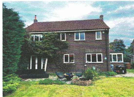
V6 - Rear view of dwelling
