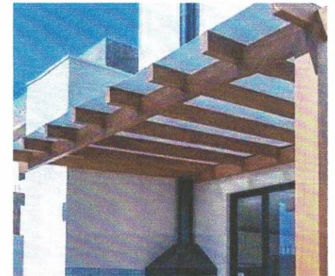
Example of timber pergola
