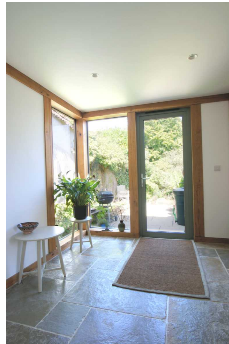
Oak framed direct glazed porch (precedent from approved extension to a GVII listed building in Dartmoor National Park (Barn End, Christow))
