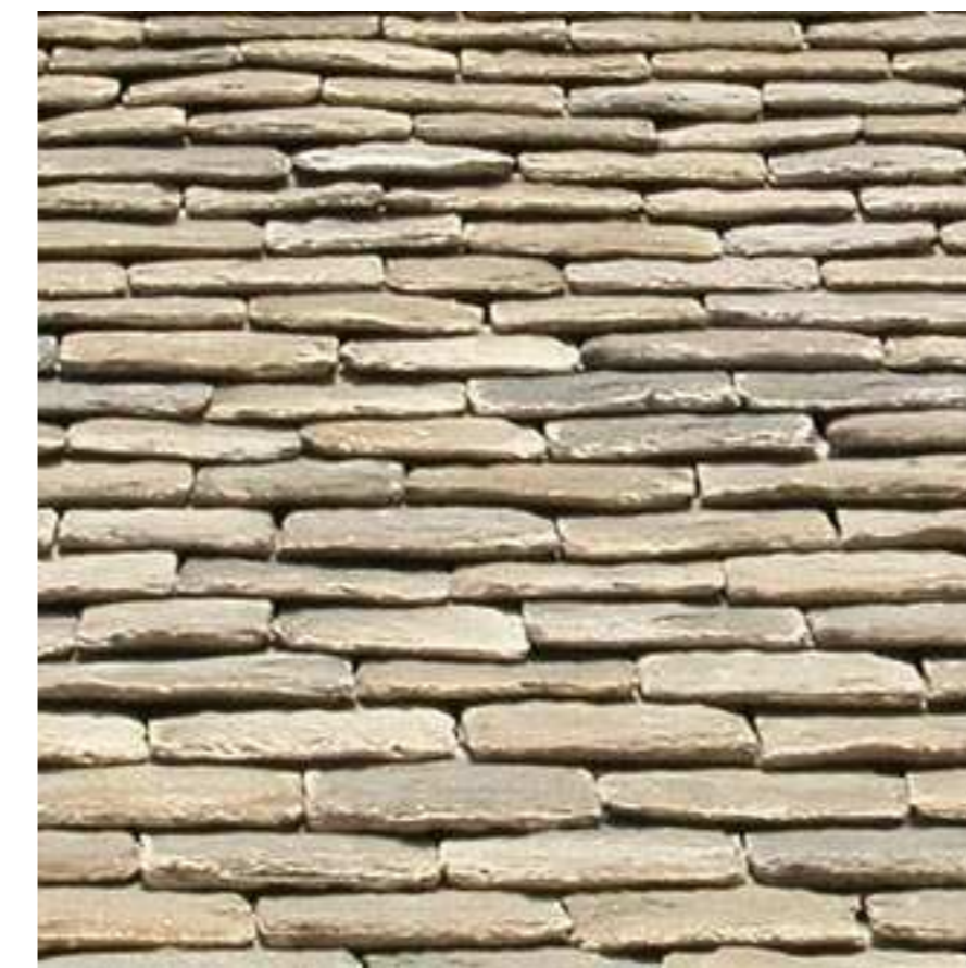
Photograph of reconstituted stone slate roof tiles laid to diminishing courses, as sample to satisfy Condition 9. Reconstituted stone slates from Cardinal Slates or similar. Not to Scale
