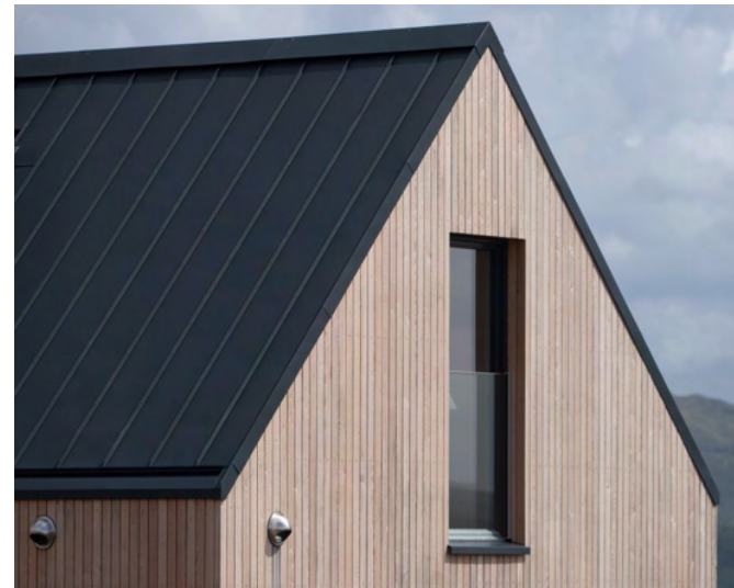
Example of zinc roof and poplar vertical cladding
