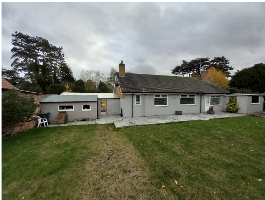
Photograph of rear elevation.
