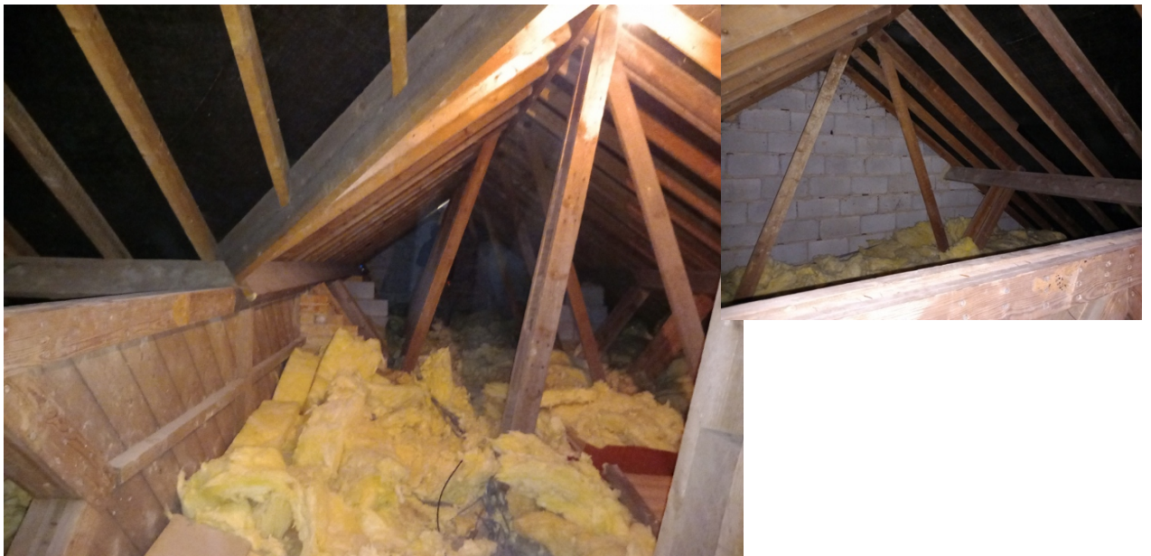
Photograph of loft space within the roof of the bungalow.
