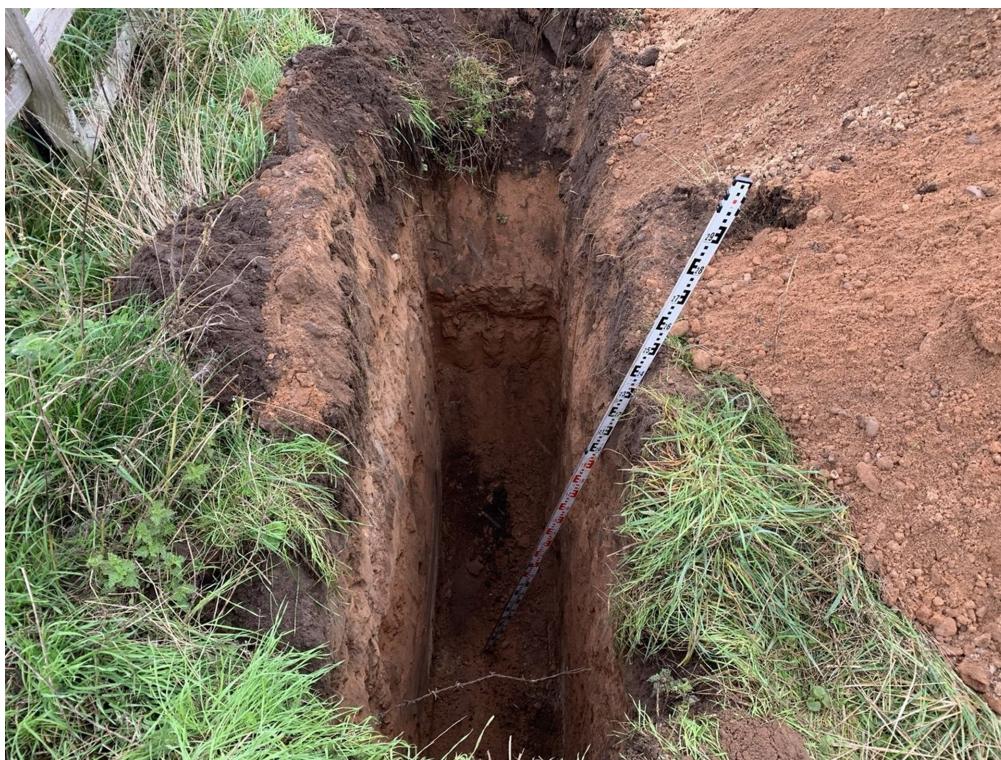
Photograph 50: TP18. Trial Pit.
