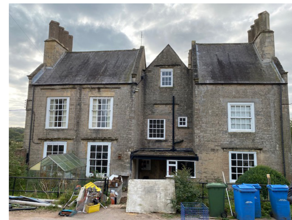
Figure 2.16 Image of rear of Carburton Manor, 2020 (Photograph; author's own)
