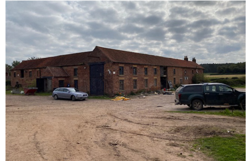
Figure 2.24 West Barns looking east (Photograph; author's own)
