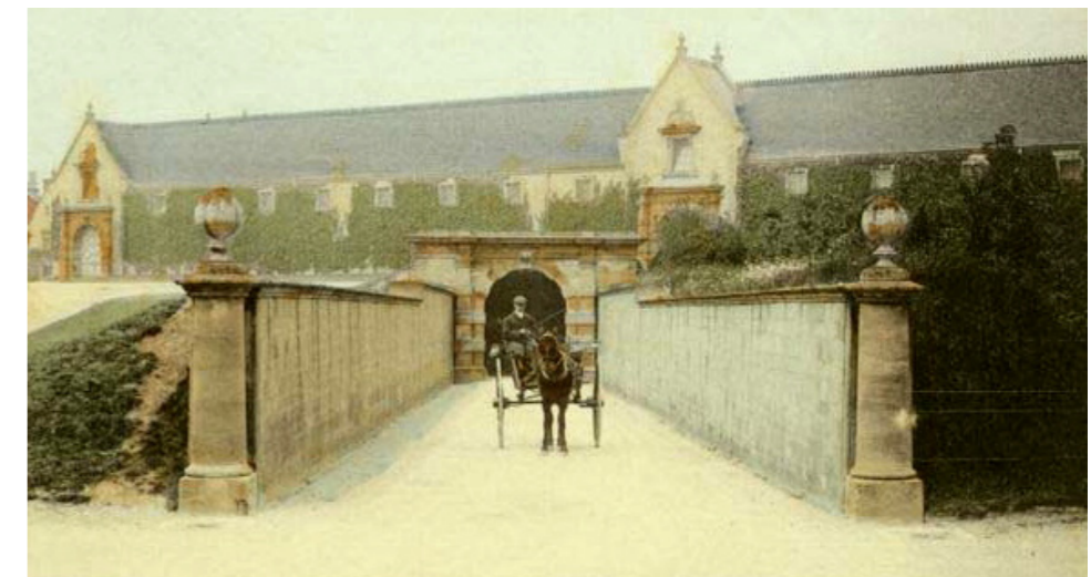
Figure 3.2 Illustration of tunnel entrance (Source : Hughie DW on www.flickr.com ).
