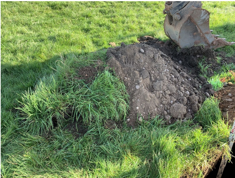
Photograph 37: TP12. Topsoil Arisings.
