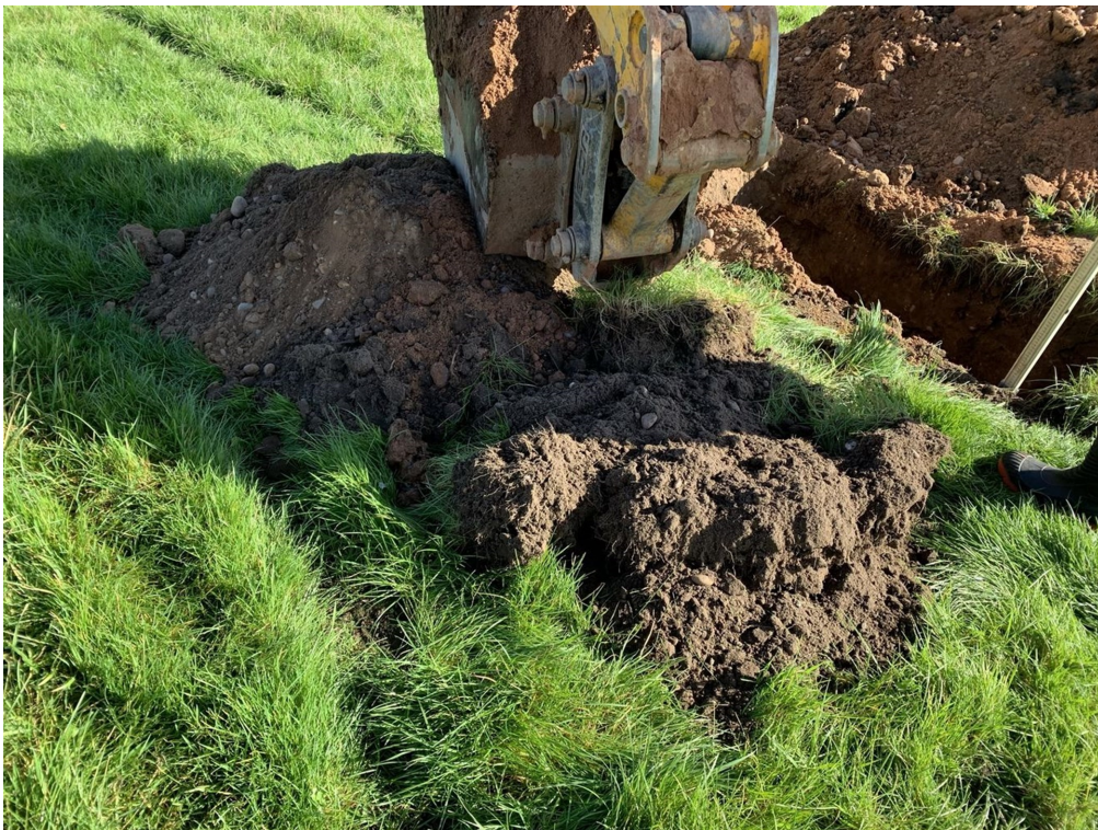
Photograph 33: TP11. Topsoil Arisings.
