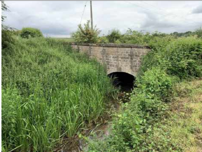
Figure 5a: Flood Dyke Field access Culvert.
