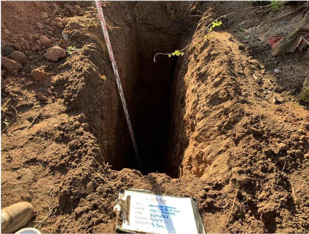
Photograph 20: TP07. Trial Pit.
