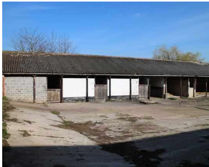
5 View looking east towards the single storey open stables.
