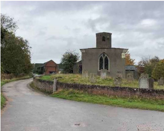
2 View east along Piper Lane
