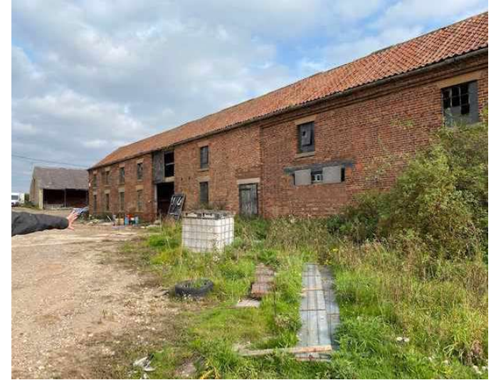
3 View looking north towards the two storey brick barns.
