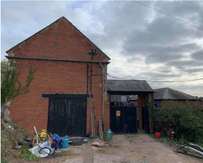
1 View looking east towards the East Barns from the Manor House.
