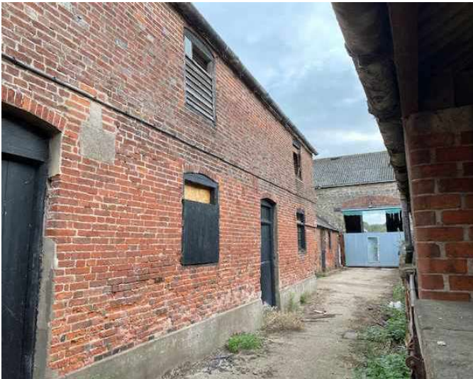
4 View looking east towards the two storey barn.
