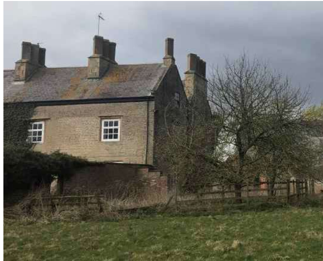
2 View looking north across the Water Meadows towards Manor House.
