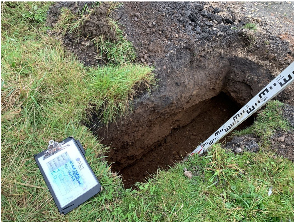
Photograph 05: TP02. Trial Pit (2).
