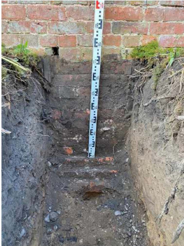
Photograph 35 – Foundation Pit 09 step
