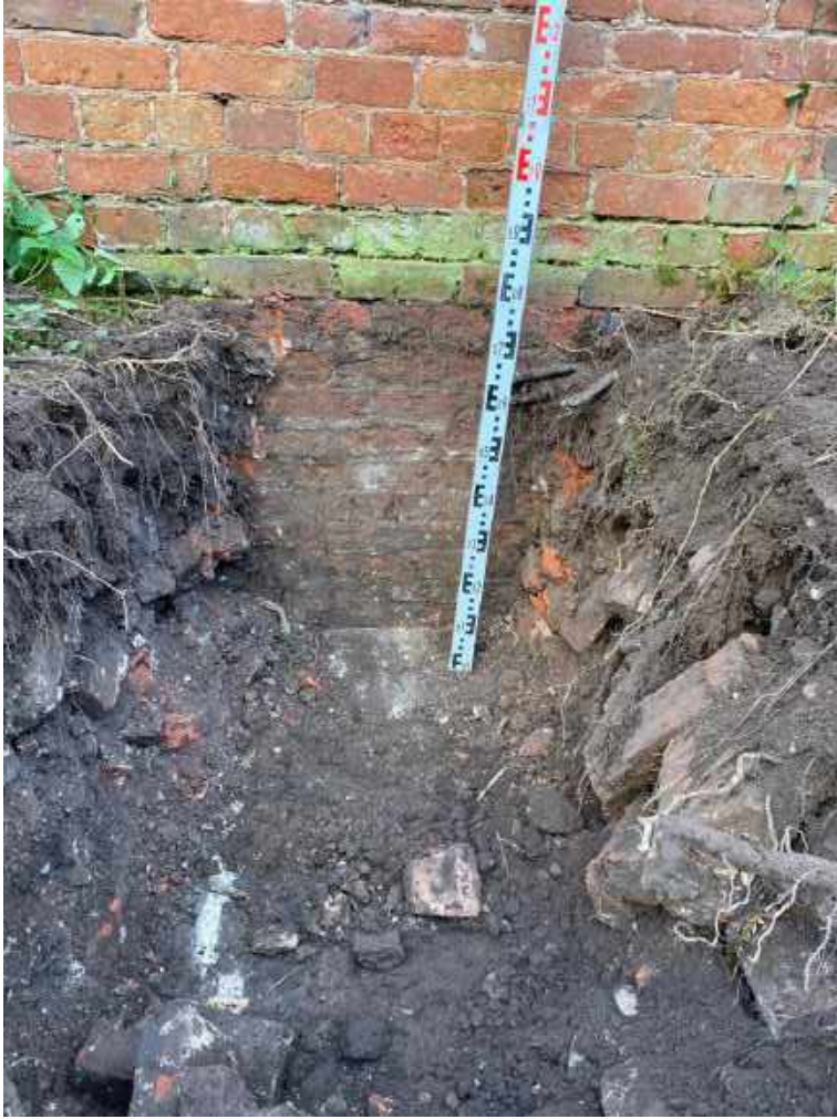
Photograph 39 – Foundation Pit 10 prior to slab being broken out
