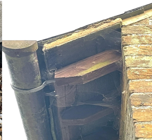
Manor Eaves Detail
