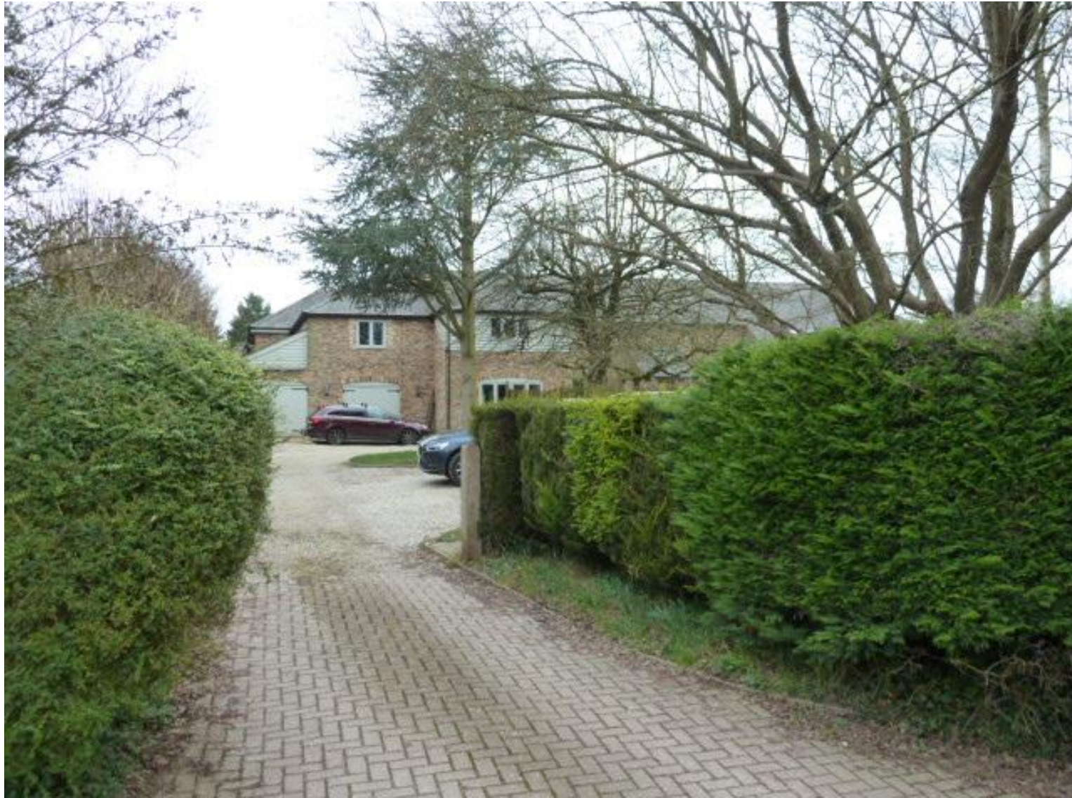
IMAGE 23 – View of 2 storey property and access, lying to the south side of Cornells Lane close to the High Street junction. It is constructed in brick, boarding and slate and benefits from vegetation around it
