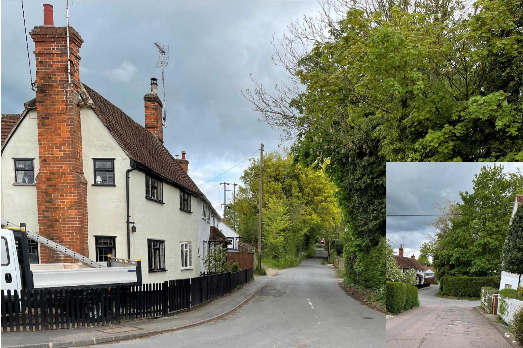
IMAGE 20 – A view east from the High Street junction looking along Cornells Lane. Corner Cottage and White Cottage (and garage) are seen to the left. The site’s maintenance access to the paddock is just visible along with the electricity power line apparatus beyond. The nearest proposed dwelling at Plot 1 would be sited c. 32m back from the existing (but to be grounded) power line apparatus. Inset Photograph is taken further west, from Hamel Way
