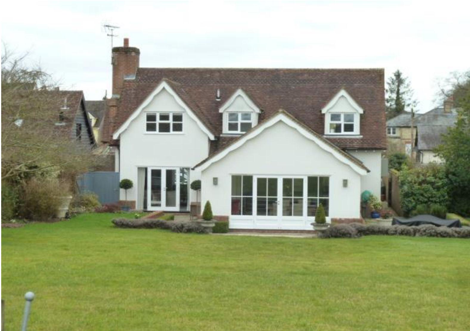
IMAGE 14 - Meadow Cottage (High Street) lies diagonally opposite the site and has an open view over part of the paddock (which will be unaffected). This 1 ½ storey property, which lies in the Conservation Area, includes a gable, dormer features, brick plinths, render chimneys and clay tiles. The property to the left (Roseley Barn) includes black boarding and clay tiles. These features and materials are used in the proposed development.
