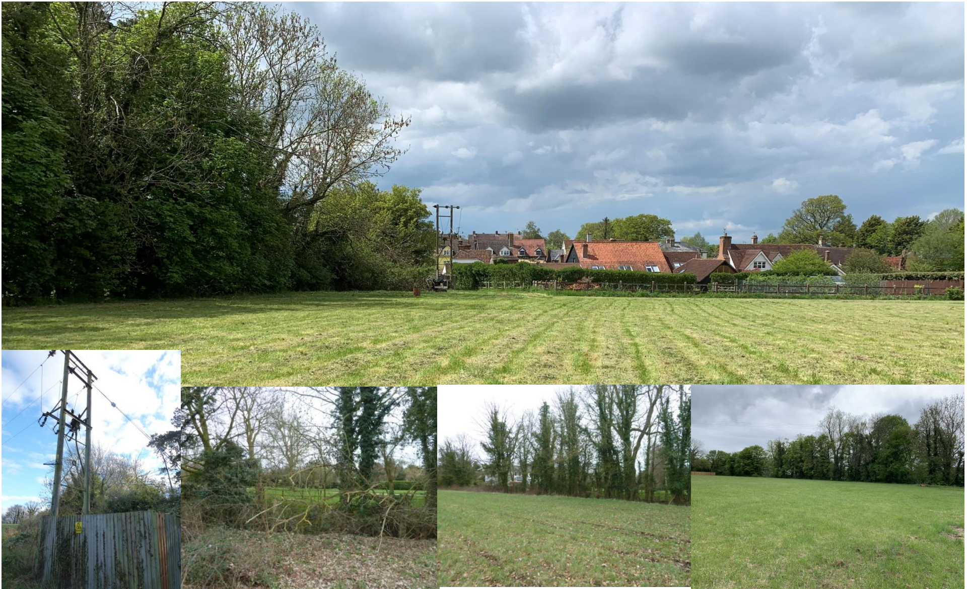
IMAGE 6 – View from in front of proposed Plot 3. A new permissive footpath will run next to the private drive in this location, opening up views of the houses lying in the conservation area (seen in the distance). Inset Images : Left - Sub station and power line apparatus; Centre Left – View across southern boundary through trees, to residential garden opposite; Centre Right & Right – eastern boundary trees looking towards Weft House.
