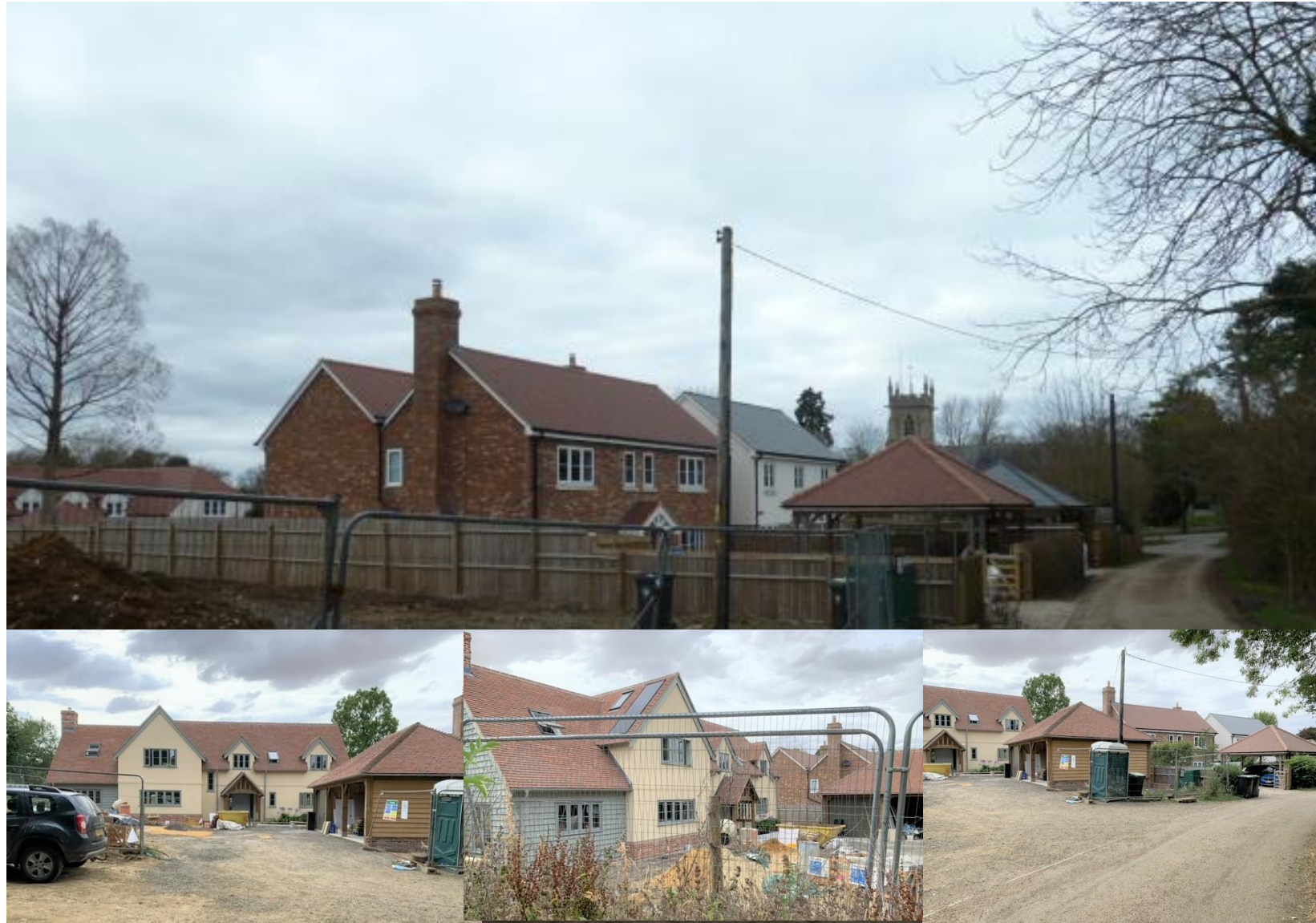
IMAGE 18 – To the west of the application site, beyond the retained paddock area, this photograph (2021) shows a modern 2 storey houses, with one in brick, with tiled roof and chimney; and another dwelling in painted render and slate roof. The upper part of Widdington Church is visible above detached ‘frontage’ cart lodges. Since this picture was taken another substantial 1 ½-1 ¾ storey dwelling of vernacular design and materials plus with detached 3 bay frontage cart lodge/garage, has been constructed to the left, as shown on the insets below, consolidating residential character of the area.
