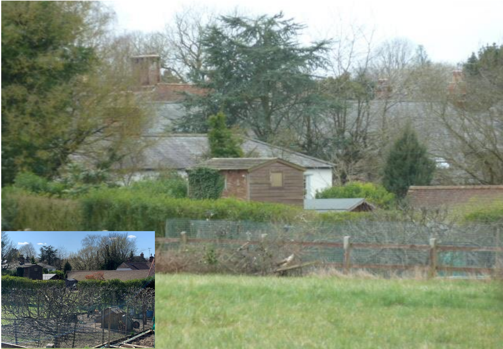
IMAGE 24 – View from retained paddock adjacent the site looking south-west showing how the setting of the listed William The Conqueror is already affected by various residential outbuildings (lying west of the site) including a tree house at Roseley Barn. Inset photograph shows similar view but closer to the application site
