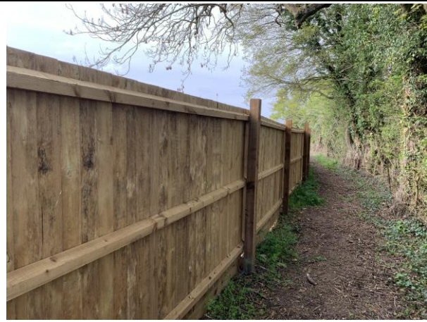
Plate 5: Close board wooden fence installed close to the eastern boundary
