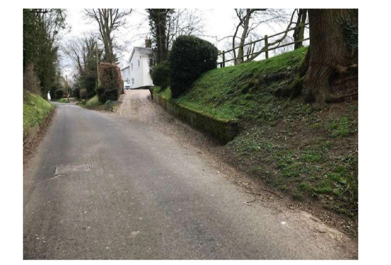
View B. Existing 9.8m wide hardened access serving Weft House.
