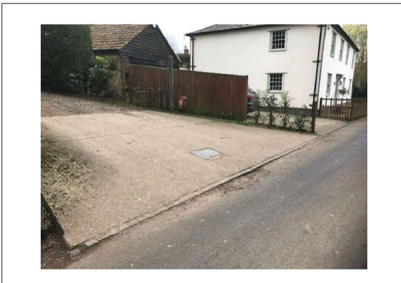
View A. Existing 13.5m wide concrete and gravel accesses serving William the Conqueror (6m wide gravel) and Weft House, Thatched (7.5m wide Concrete).
