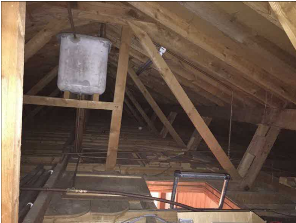
Photo 4. Roof void of building showing wood lining
