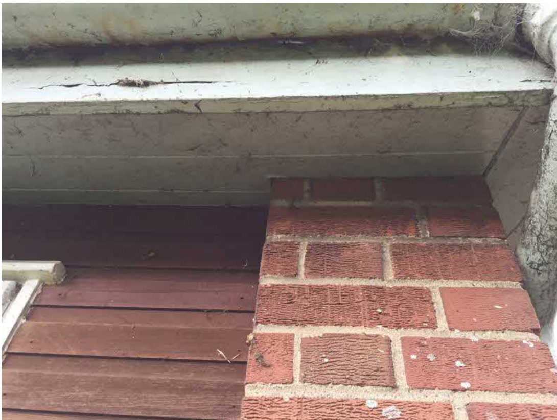
Photo 16: Rotten soffit
