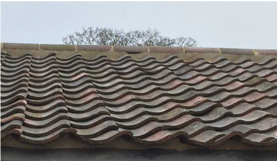
Photo 20. Example of a bat-accessible ridge tile on a pantile roof
