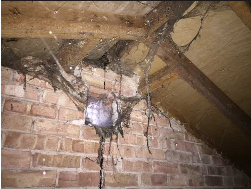
Photo 5. Example of cobwebbed air vents to north and south
