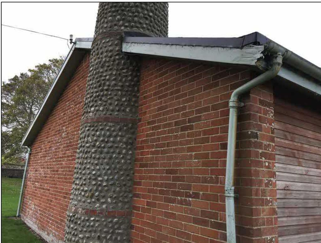
Photo 8. South elevation showing cobble-clad chimney
