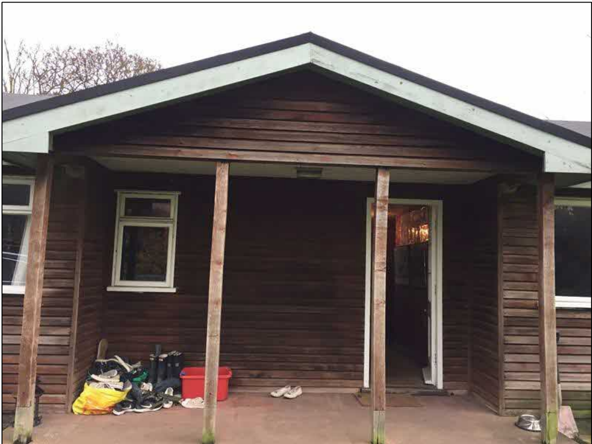
Photo 2. Porch on west side of dwelling
