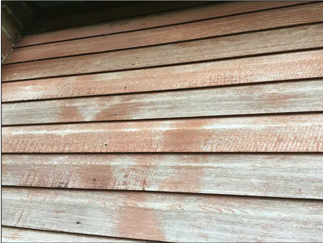
Photo 3. Example of cladding on west and east elevation
