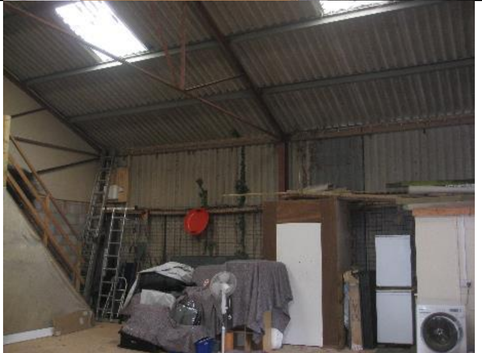
Photo 4: Building B1 uninsulated storage area at east end of building with skylights giving good illumination in day time.
