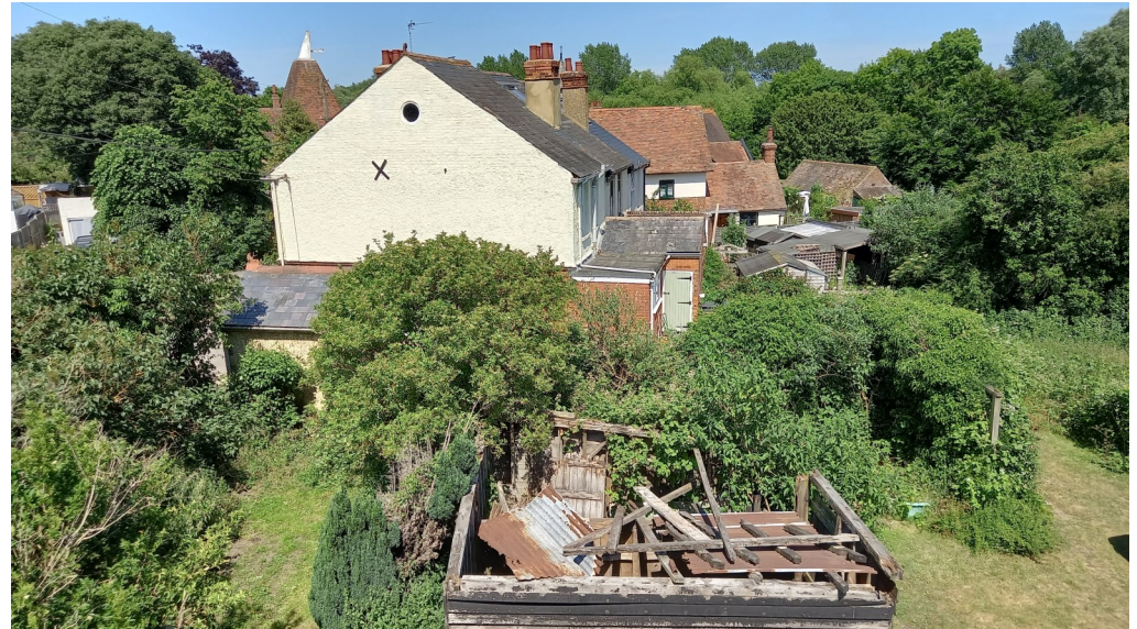
view of stables from house looking east towards New Cottages
