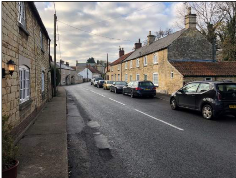
05. View south along High Street from the front of the site.
