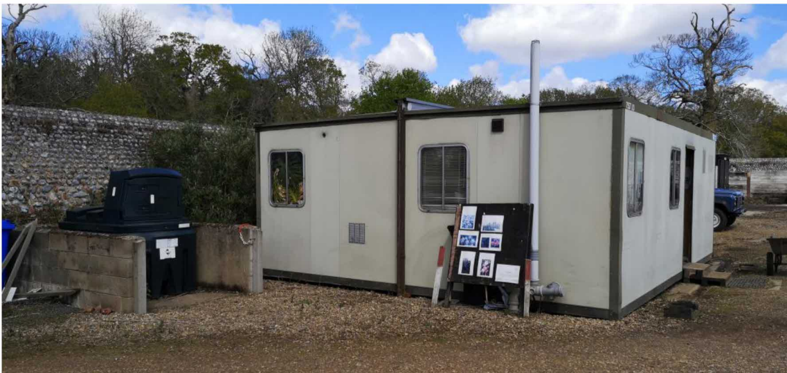
Fig.5: View of the South elevation of the existing bothy.
