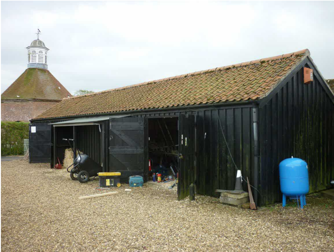
Fig.6: View looking East of the garden storage building running along the South side of the Gardener's Yard.
