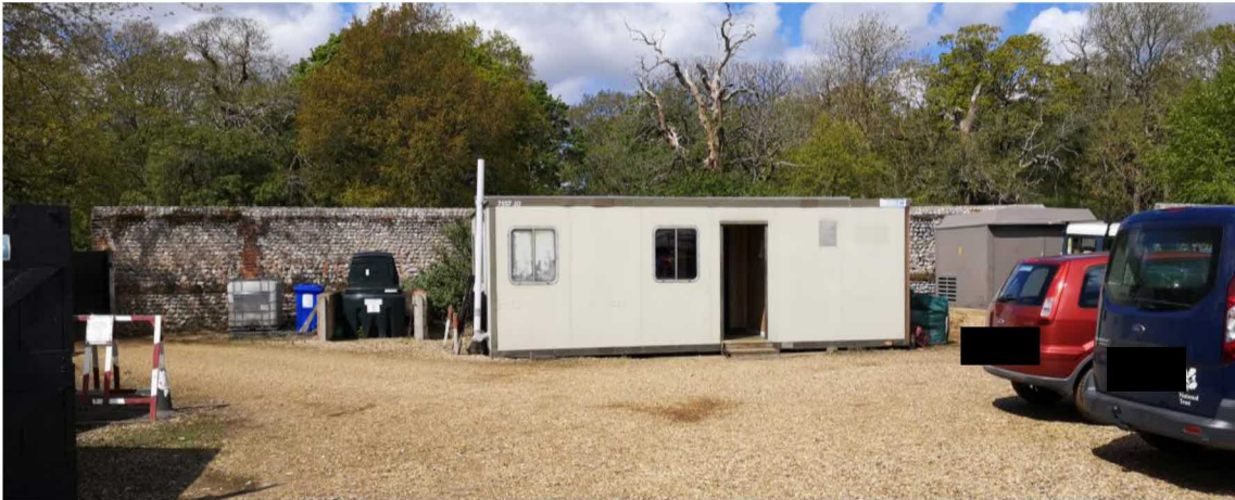
Fig.3: View of the East elevation of the existing bothy.
