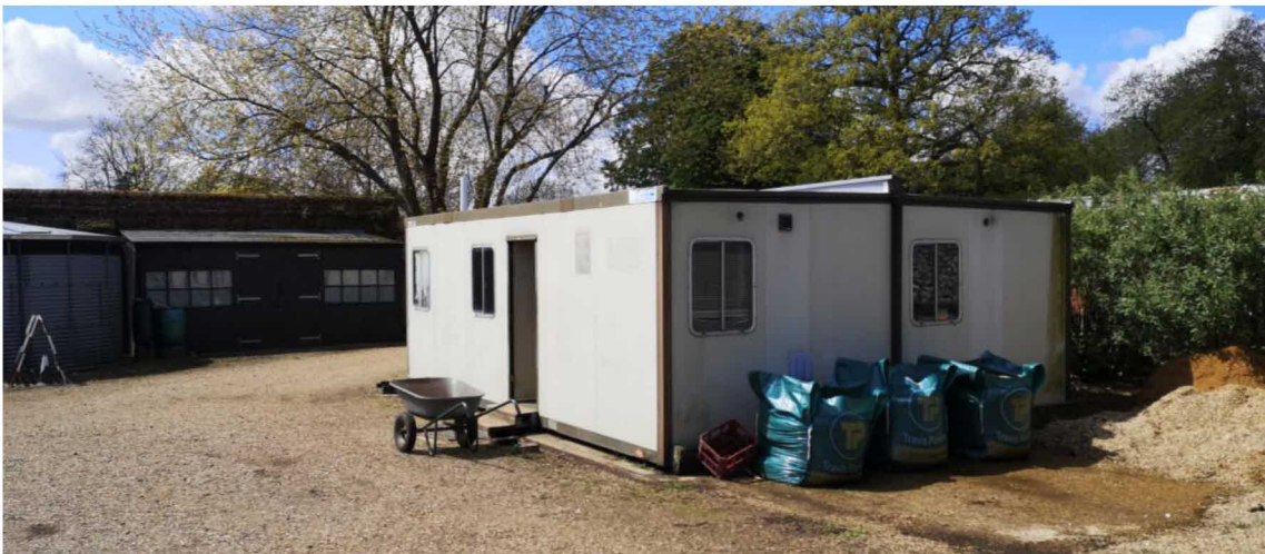
Fig.4: View looking South showing the North and East elevations of the existing bothy.
