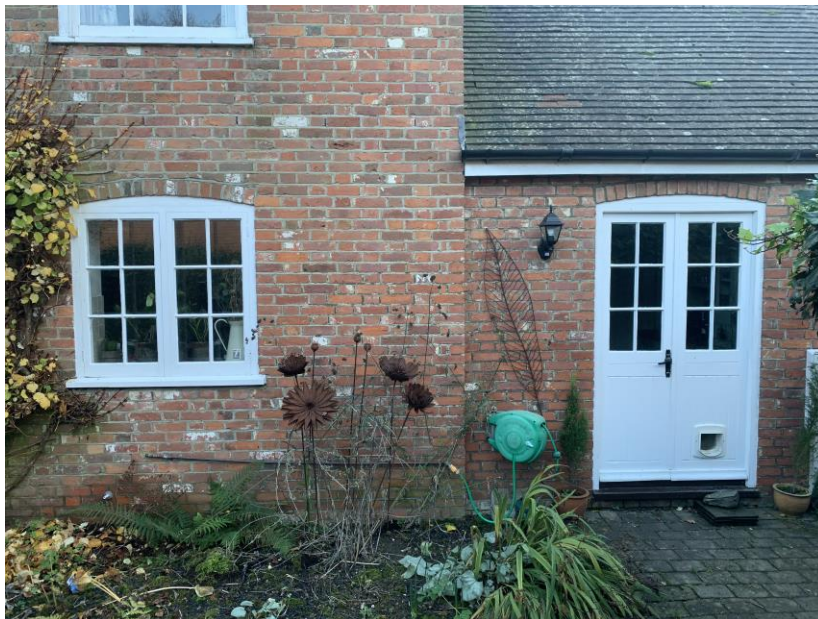
Front of the house showing the unused kitchen doors to be replaced with another kitchen window the same as the existing window seen here to the left
