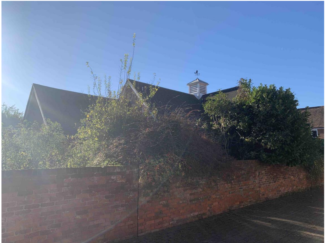
Front of the house from the eastern end of the courtyard
