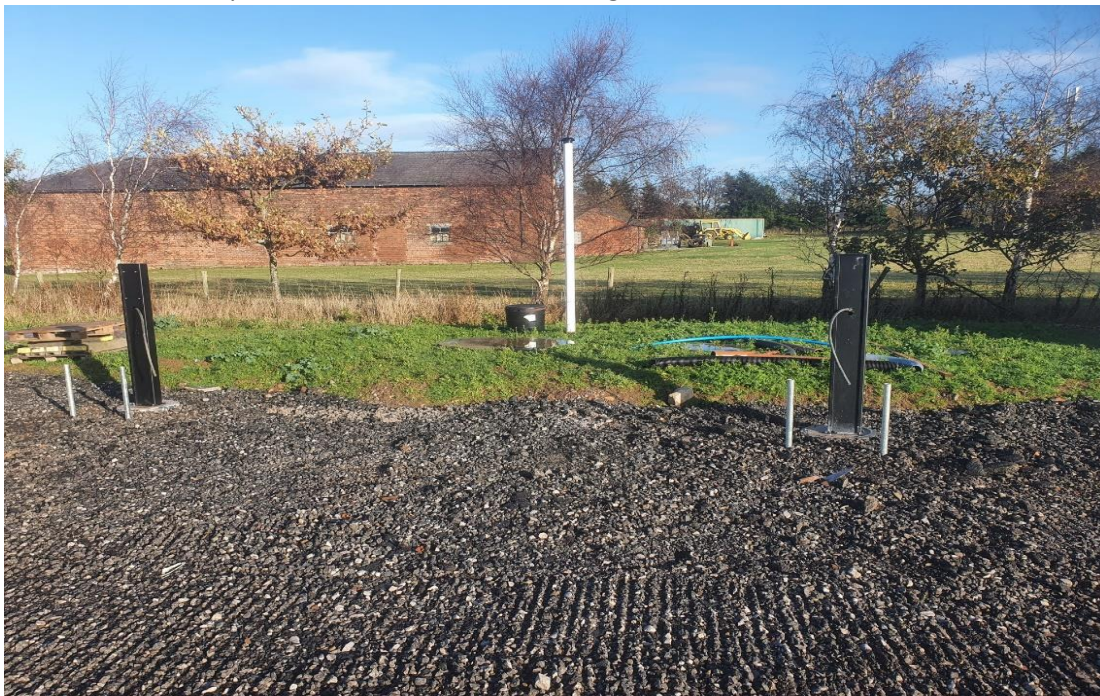
Figure 1 Two mounting poles for EV charger with electric cable in place
