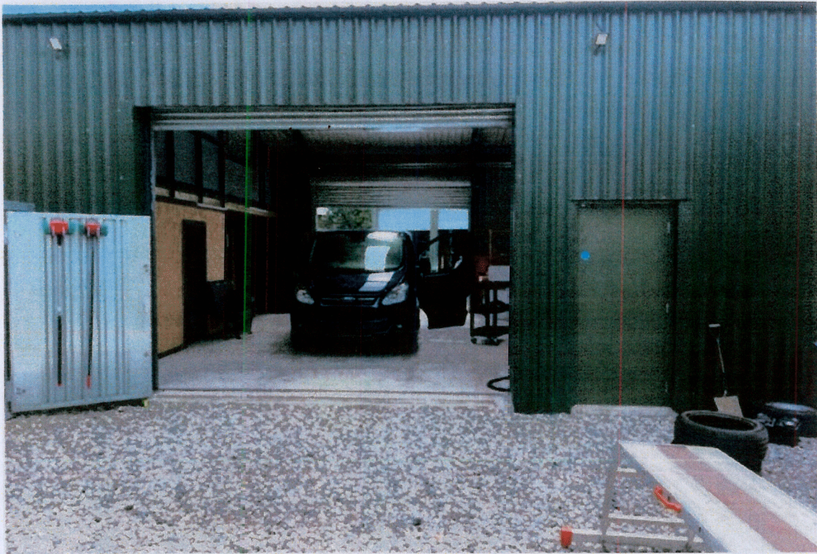
PHOTO 3. Shows the rear. Exit door and parking area
