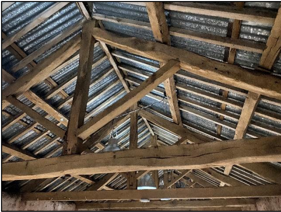
Plate 3: Underside of barn roof
