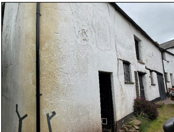
Plate 1: Front of barn (facing south-east)
