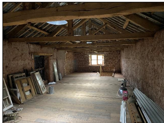
Plate 2: First floor of barn (facing north)
