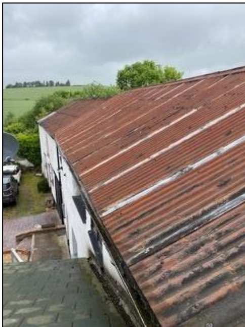
Plate 5: External view of roof (facing north)
