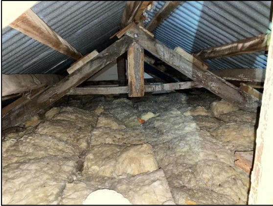
Plate 6: Roof void above living space (facing south)
