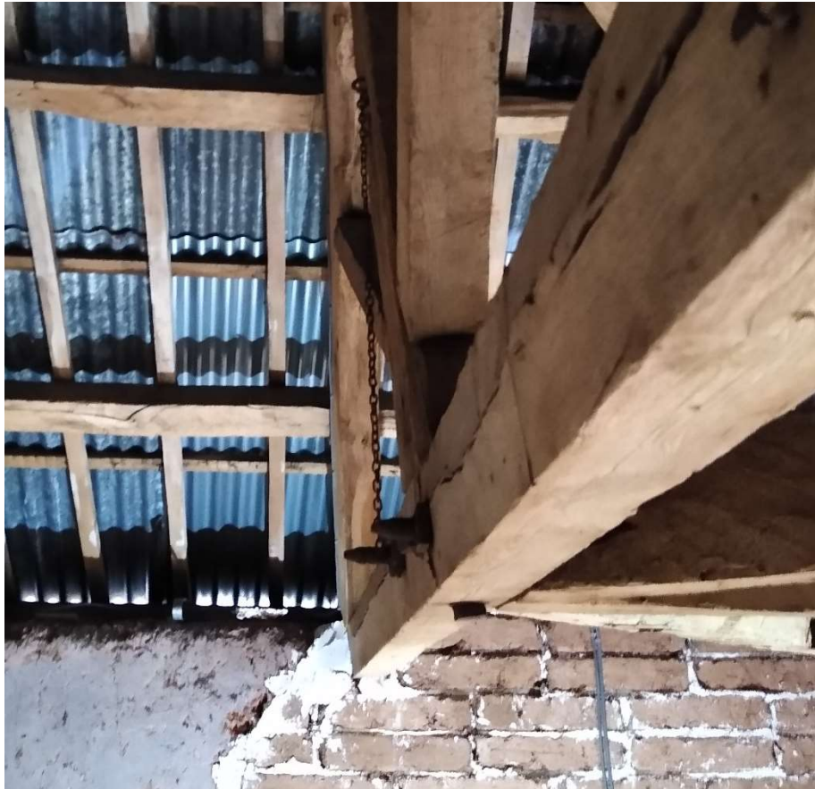
Image 2 - West bearing north truss
