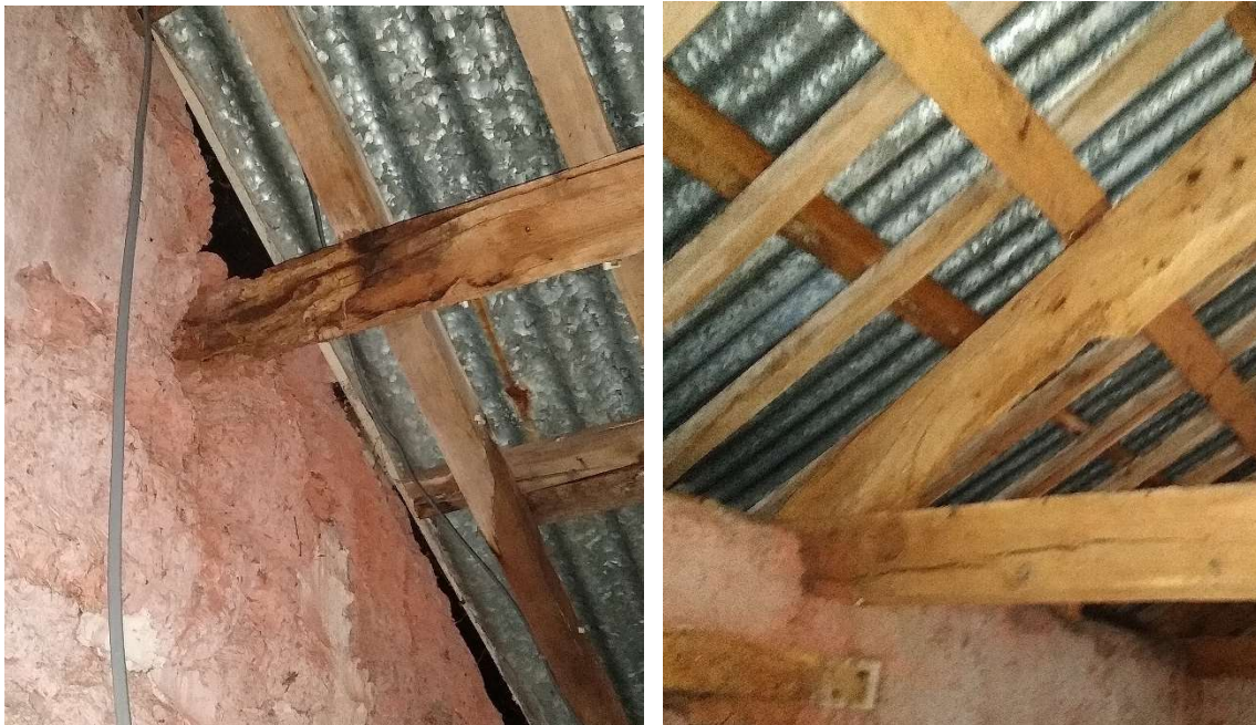
Image 3 - South end truss and west purlin
