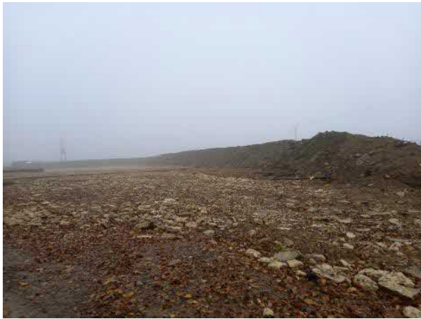
Plate 1: Bare earth and rubble at southern end of area for proposed padel courts, with boundary earth bund.
