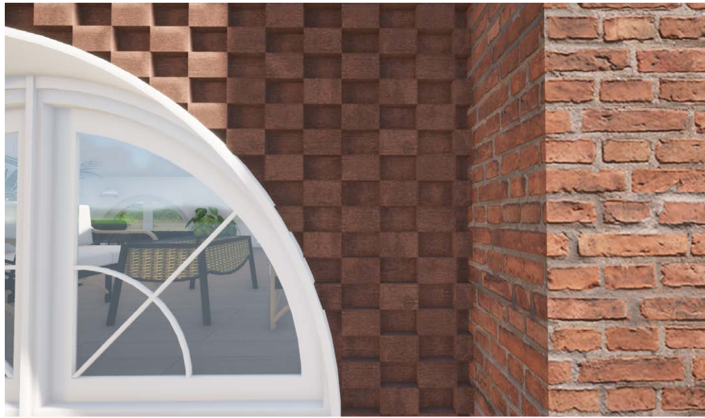
Render of proposed 'hit & miss' brick detail
