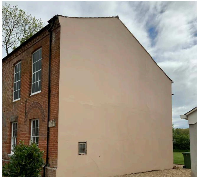
V3 - View looking South at the North side of the 'Gap'
