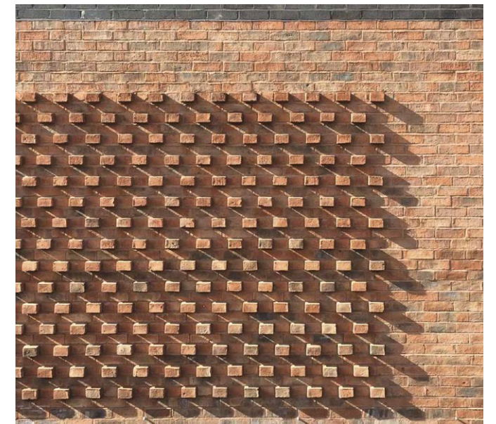
Reference image showing projecting brick headers
