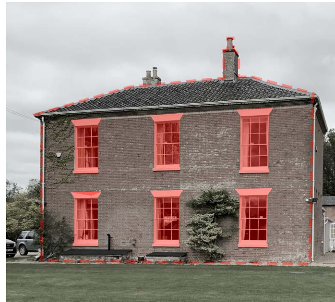
V1 - Sash windows - Glazing bars beneath skewback arches
