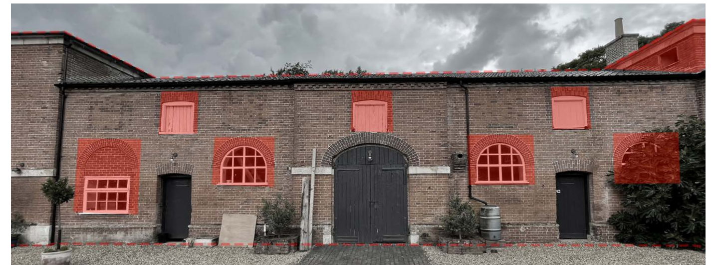
V5 - Semicircular headed ground floor openings - small windows to upper floor with cambered soffits
