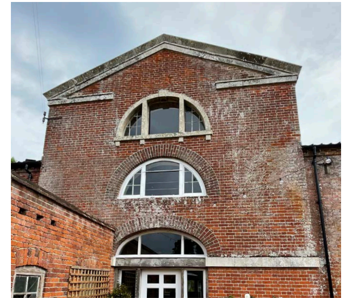
V1 - View of diocletian windows to Stable block
