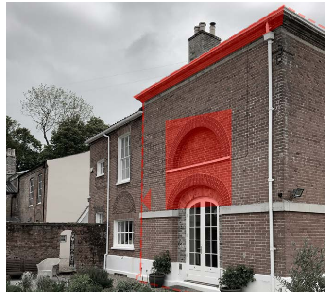
V2 - Projected facade - blind 3-centred arch with a blind lunette above
