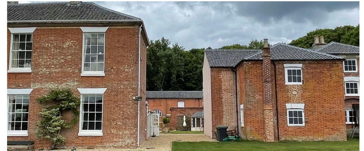
Existing view looking West
