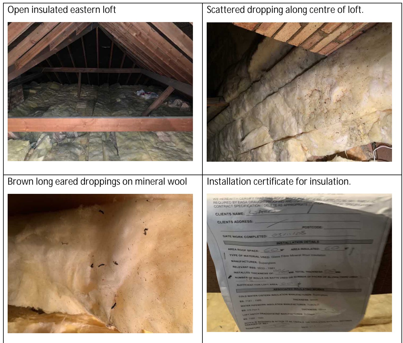
Figure 4.3 Internal survey photographs of eastern loft section.
