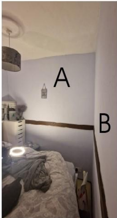
View of wall A and B.
