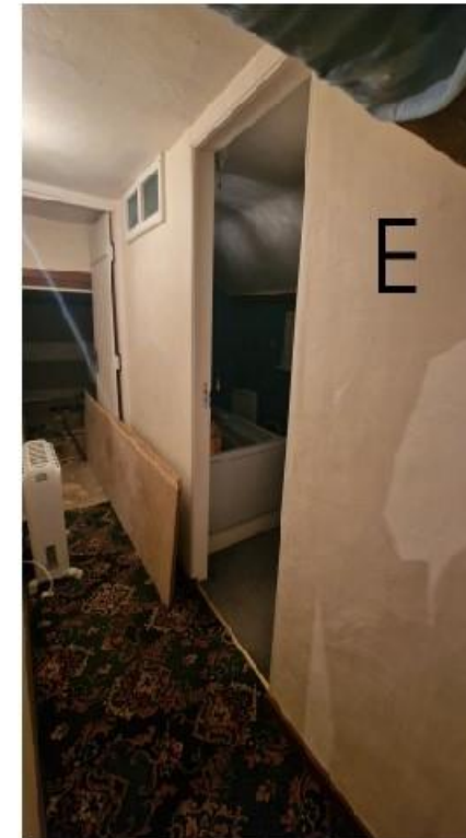
View of wall E. Plasterboard over studs
