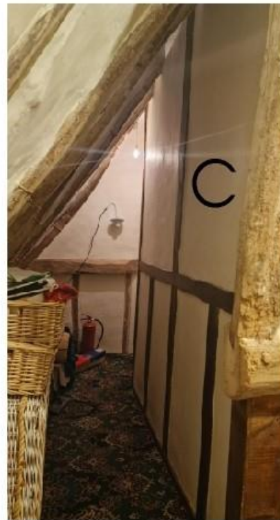
View of wall C. Plasterboard over studs softwood trim
