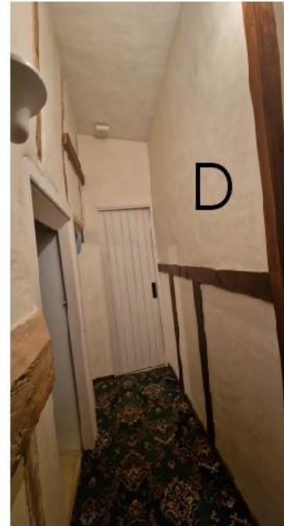
View of wall D. Plasterboard over studs softwood trim
