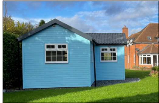
Southern Elevation of Shed
