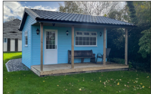
Northern Elevation of Shed
