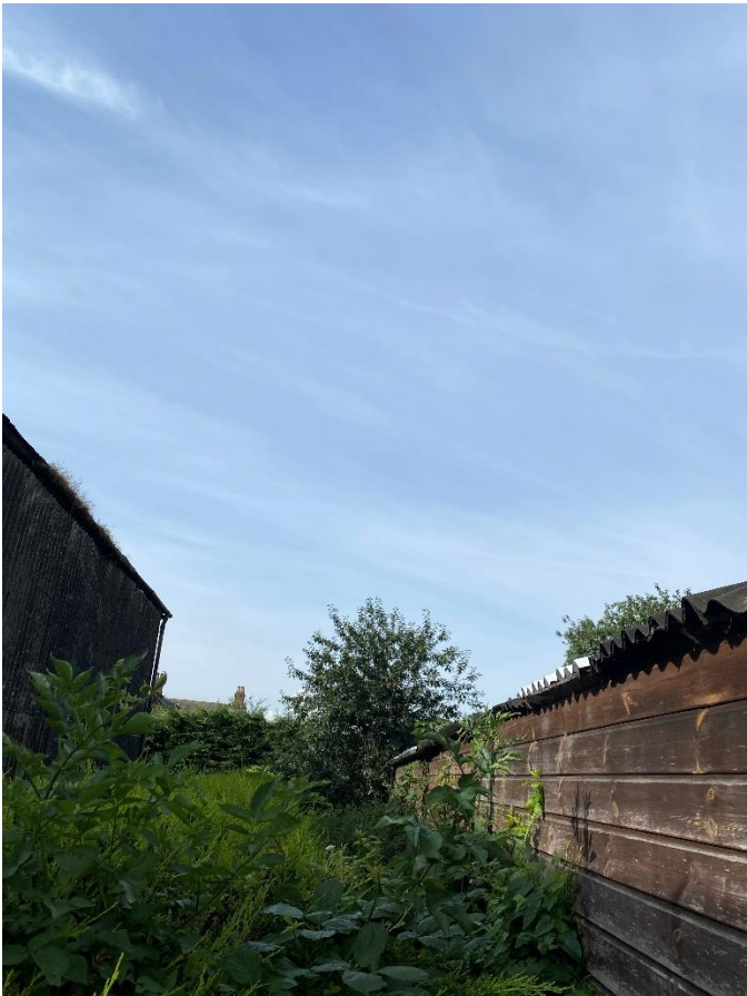
Plate 2 – The south-eastern aspect of the building
