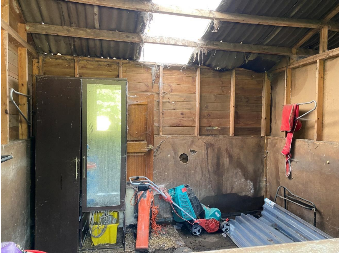
Plate 6 – Internal character of stable
