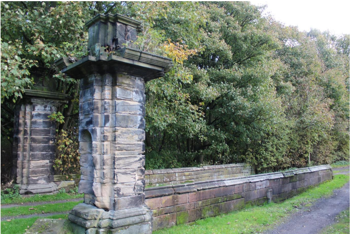
Plate 10 – Gate Piers & Bridge
