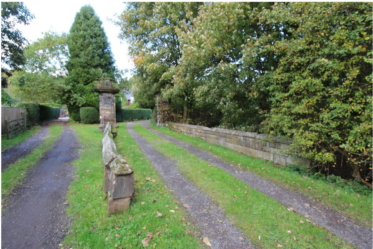
Plate 8 – Gate Piers & Bridge
