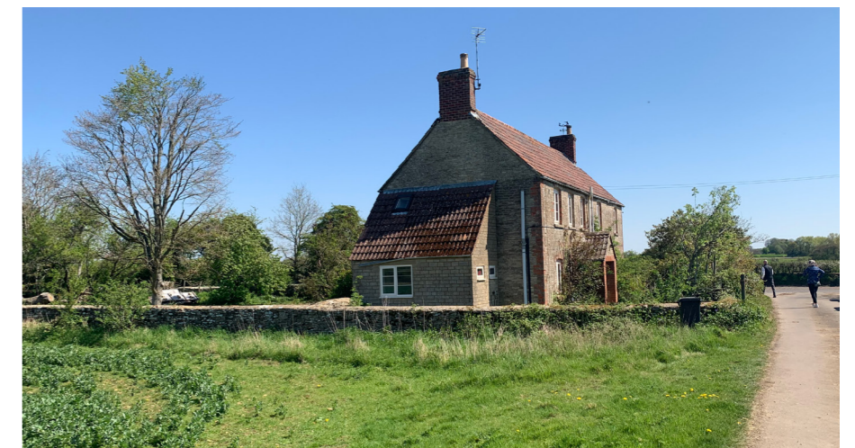
View of West Elevation from within the garden
