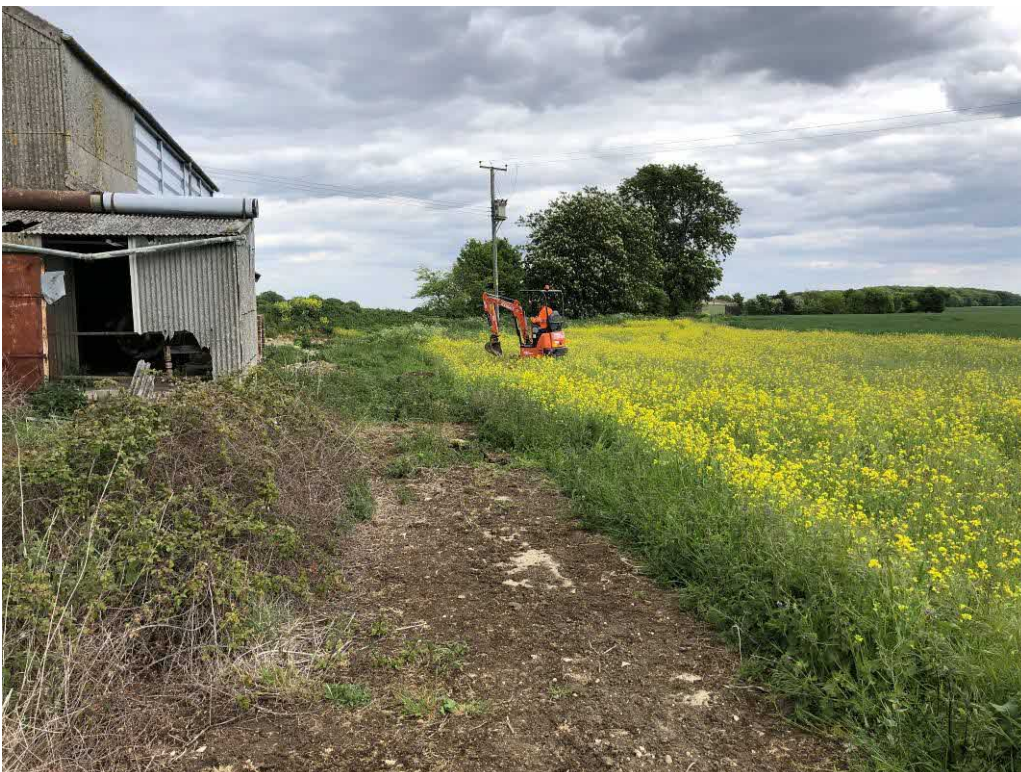
Photograph 18 – Shallow trial pitting along field boundary for evidence of asbestos fragments
