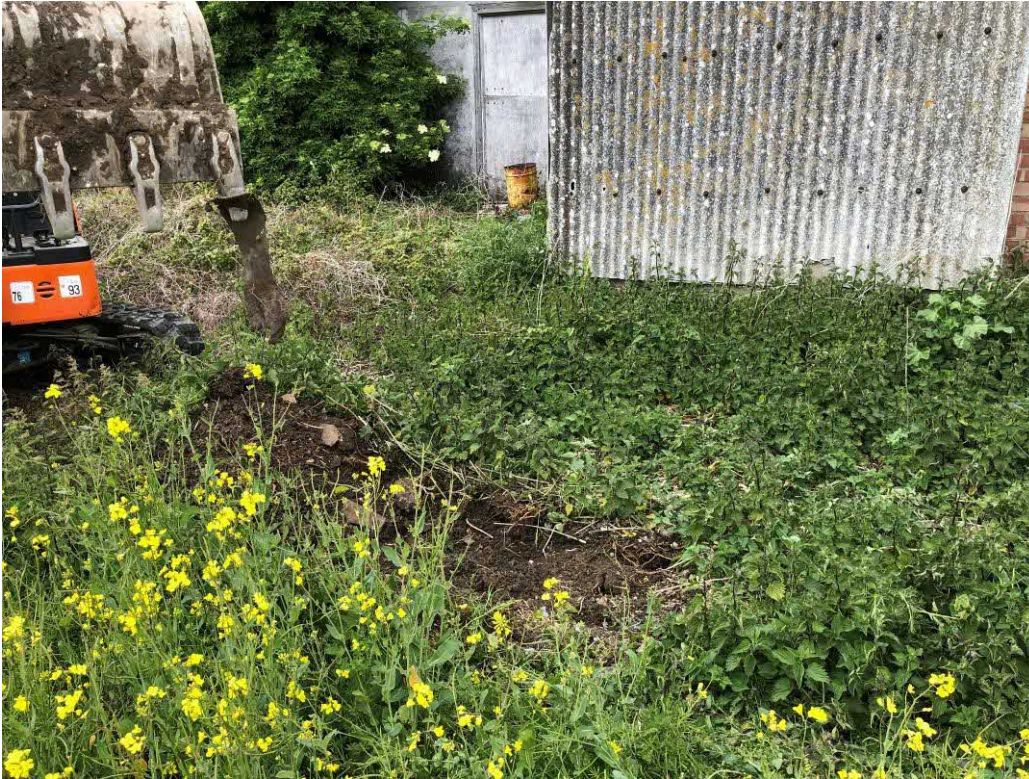
Photograph 18 – Shallow trial pitting along field boundary for evidence of asbestos fragments
