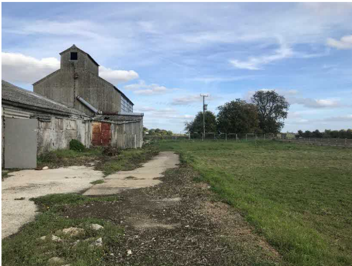
Figure 6: October 2022 - View looking east across the back of the barn. Vegetation has been cut back and drum and broken asbestos sheeting cleared.
