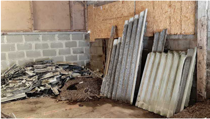
Figure 11: October 2022- Internal view of barn showing the stored broken asbestos sheeting.
