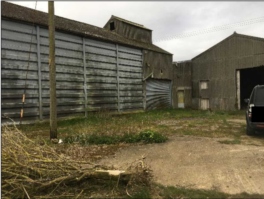
Yard Area in Front of Main Structures
