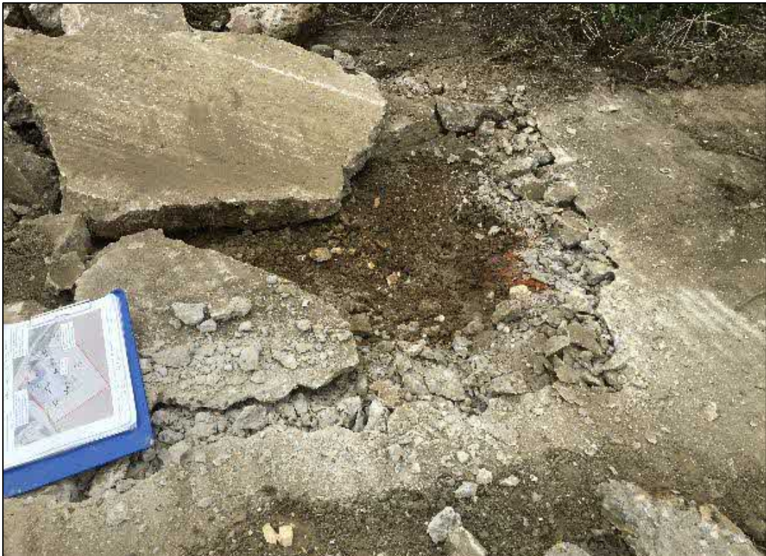
Trial pit through Concrete Apron to rear of Main Structure (TP108)
