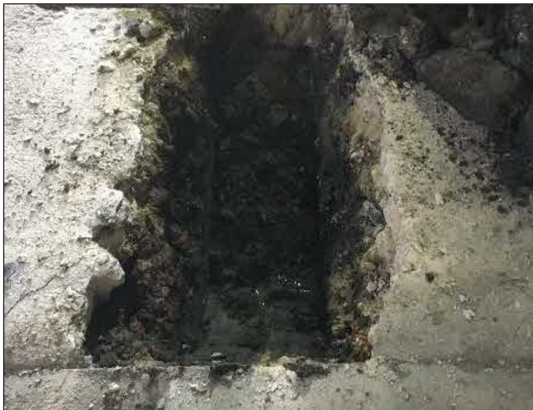
Trial pit through Concrete Slab under Main Structure (TP109)
