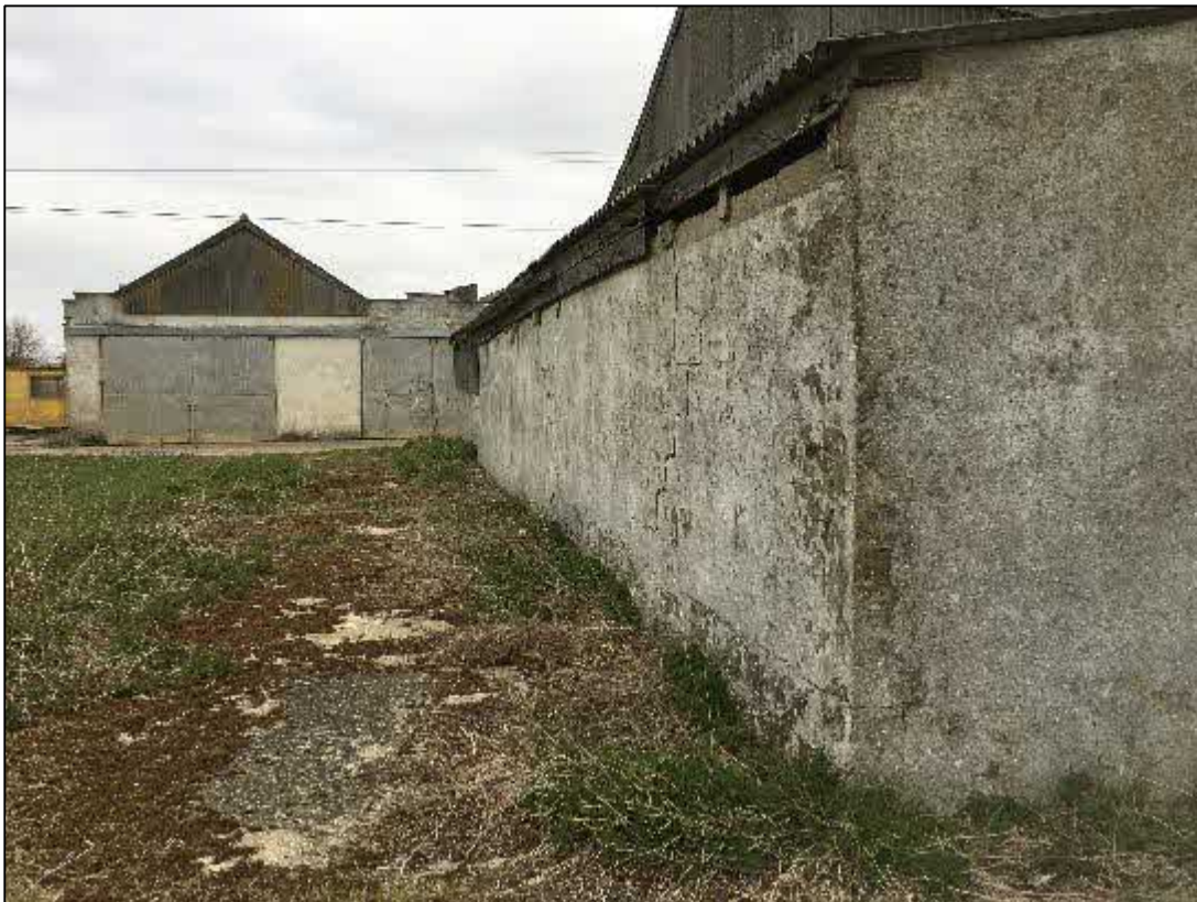
Concrete Apron to West of Main Structure
