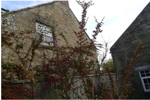
Window to the west elevation of Glebe House
