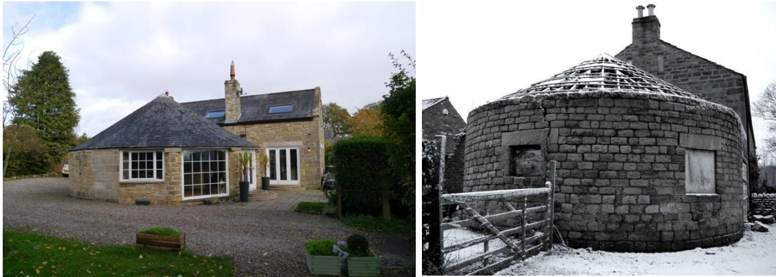
(Left) The site, and (right) a further example of a 'Gin Gan' structure (image courtesy of Wikipedia)
