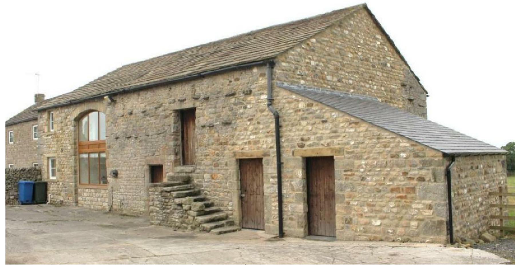
IMAGE TO SHOW EXCEPTIONAL CONDITION OF THE BARN
