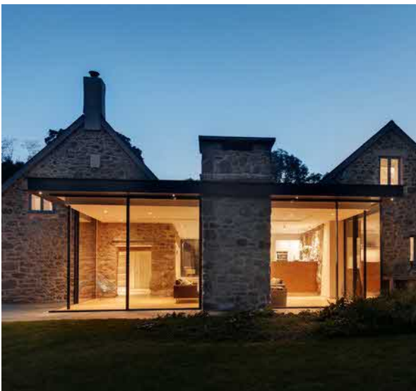
The door and windows to the ground floor extension is proposed to be slim framed black aluminium framed glazing.
