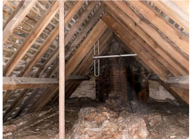
North section of roof space
