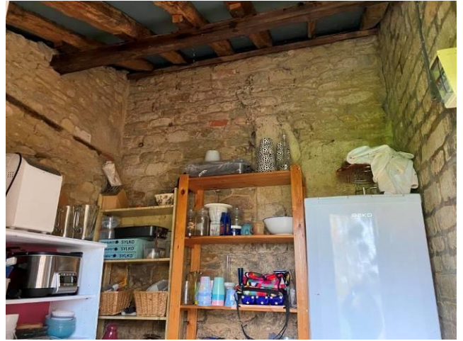
Interior of northern outbuilding to south of farmhouse
