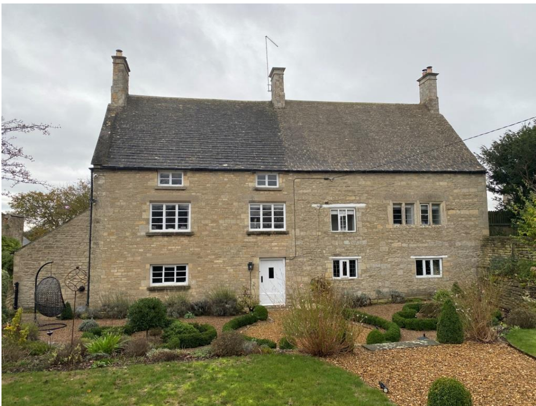
West elevation of farmhouse
