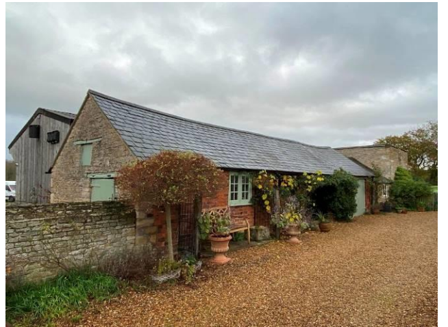
South and west elevations of western outbuildings
