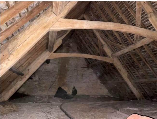
South section of roof space
