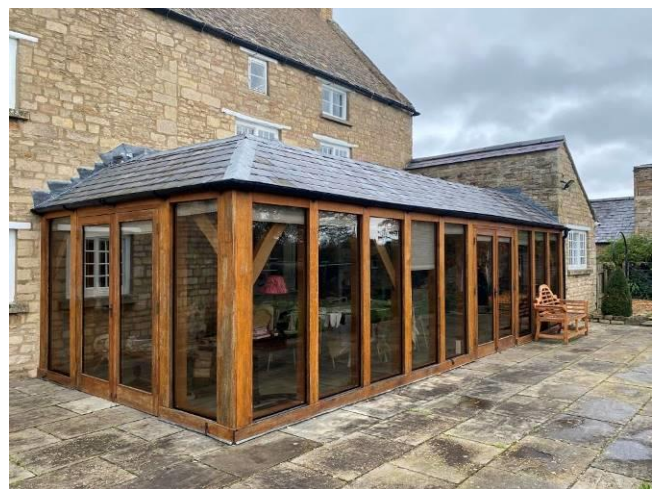
South and east elevations of glazed extension
