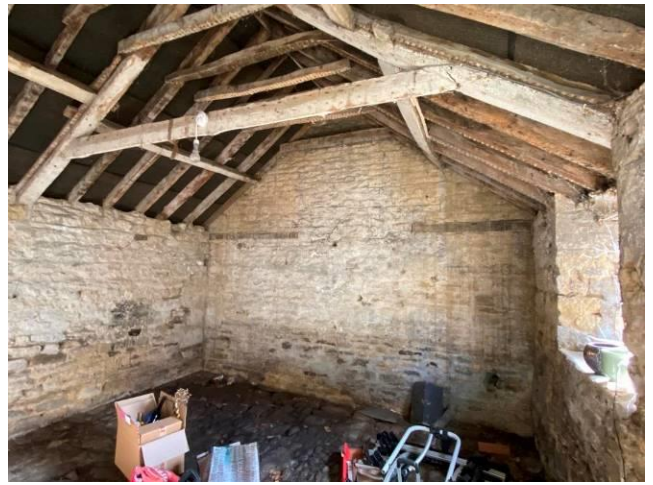
Store in central section of western outbuildings
