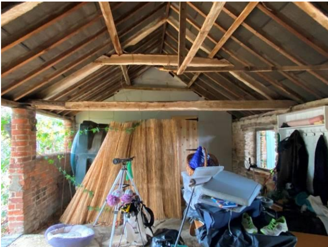
Store in central section of western outbuildings
