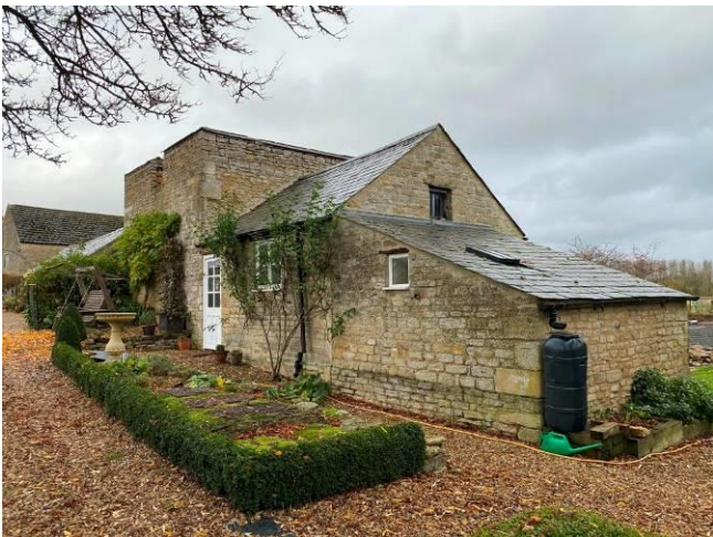
South and east elevation of eastern outbuildings
