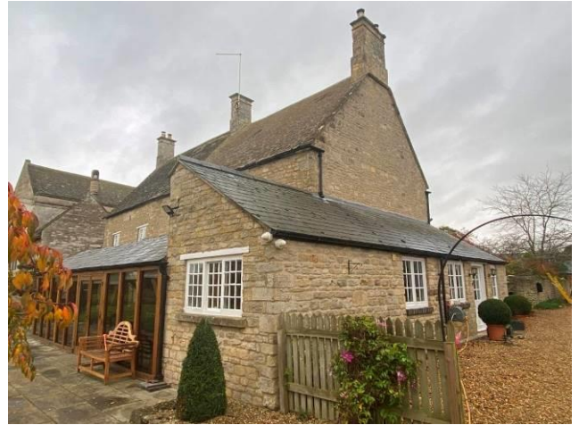
North and east elevations of farmhouse and extension
