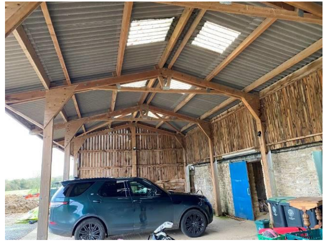
Interior of car port
