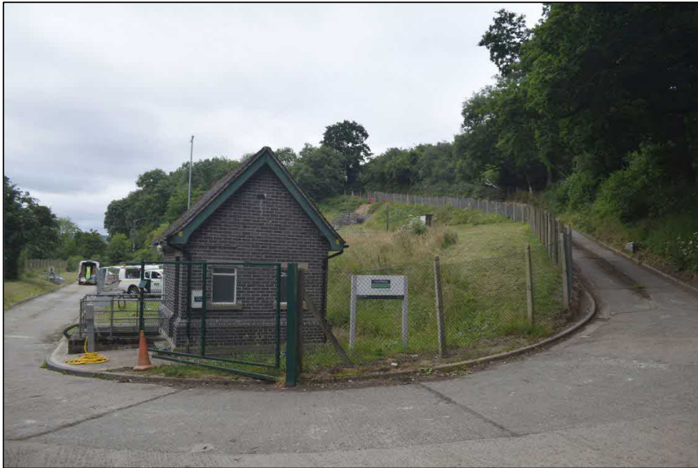
Fig. 6 Sewage treatment works viewed from the north CPAT Photo 5001-001
