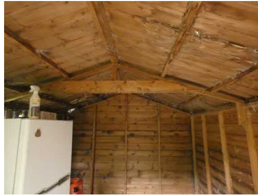
Fig. 15 Interior of shed
