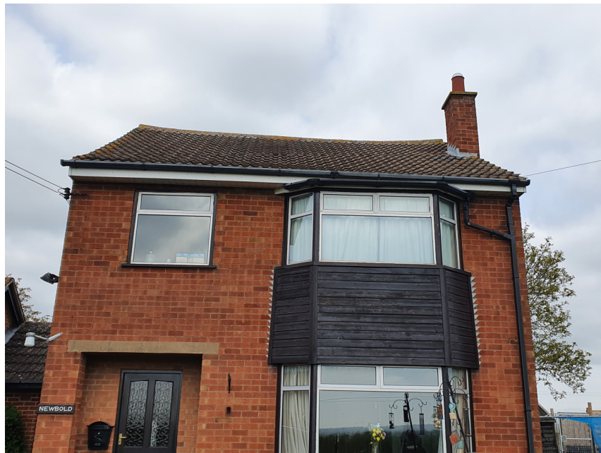
Photograph 3 - Southern aspect of dwelling
