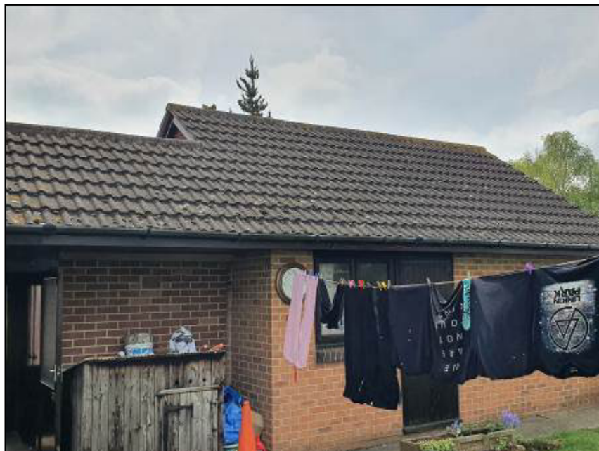
Photograph 5 - Northern aspect of garage and walkthrough
