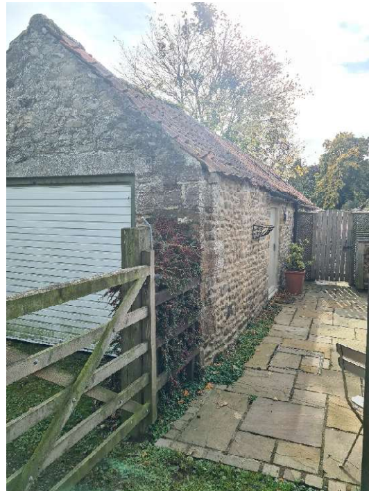
FIG.08 - Outbuildings to Other Properties on Grange terrace
