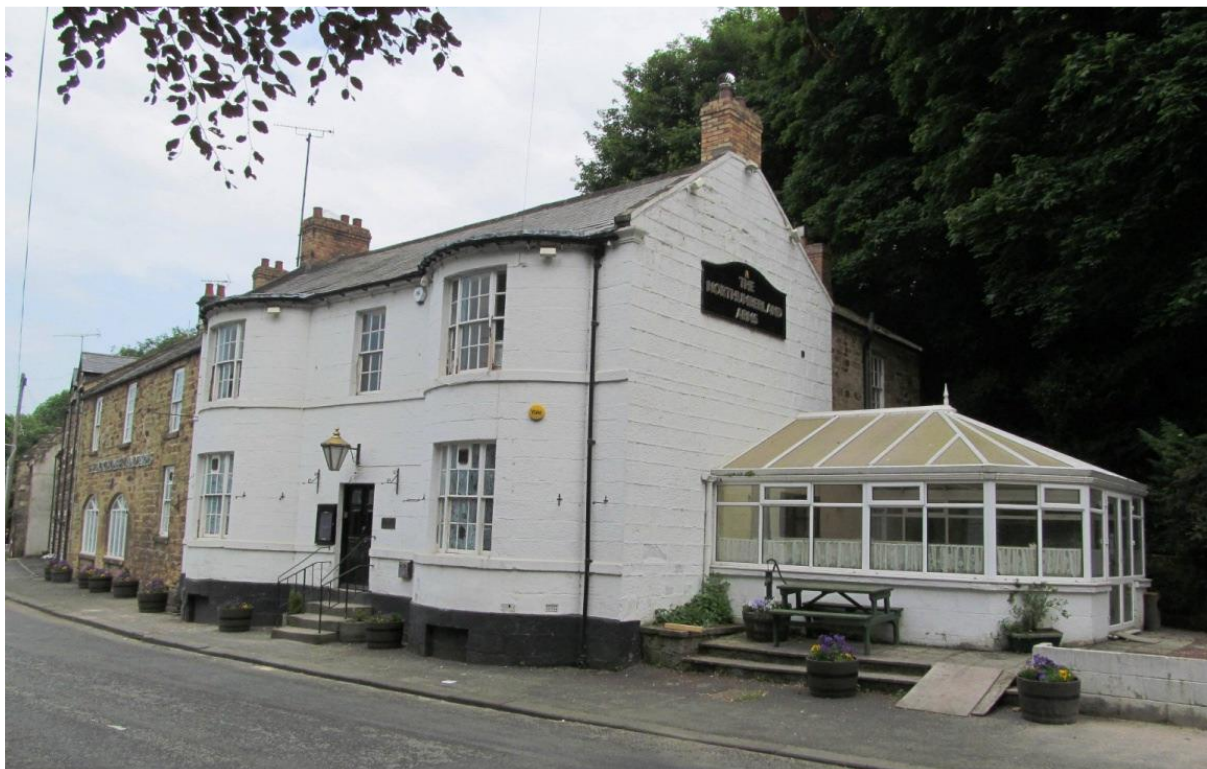
Image 5: Now whitewashed with uPVC conservatory extension – erected 1990
