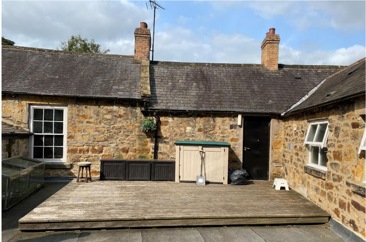
Image 14: Existing roof between bedrooms
