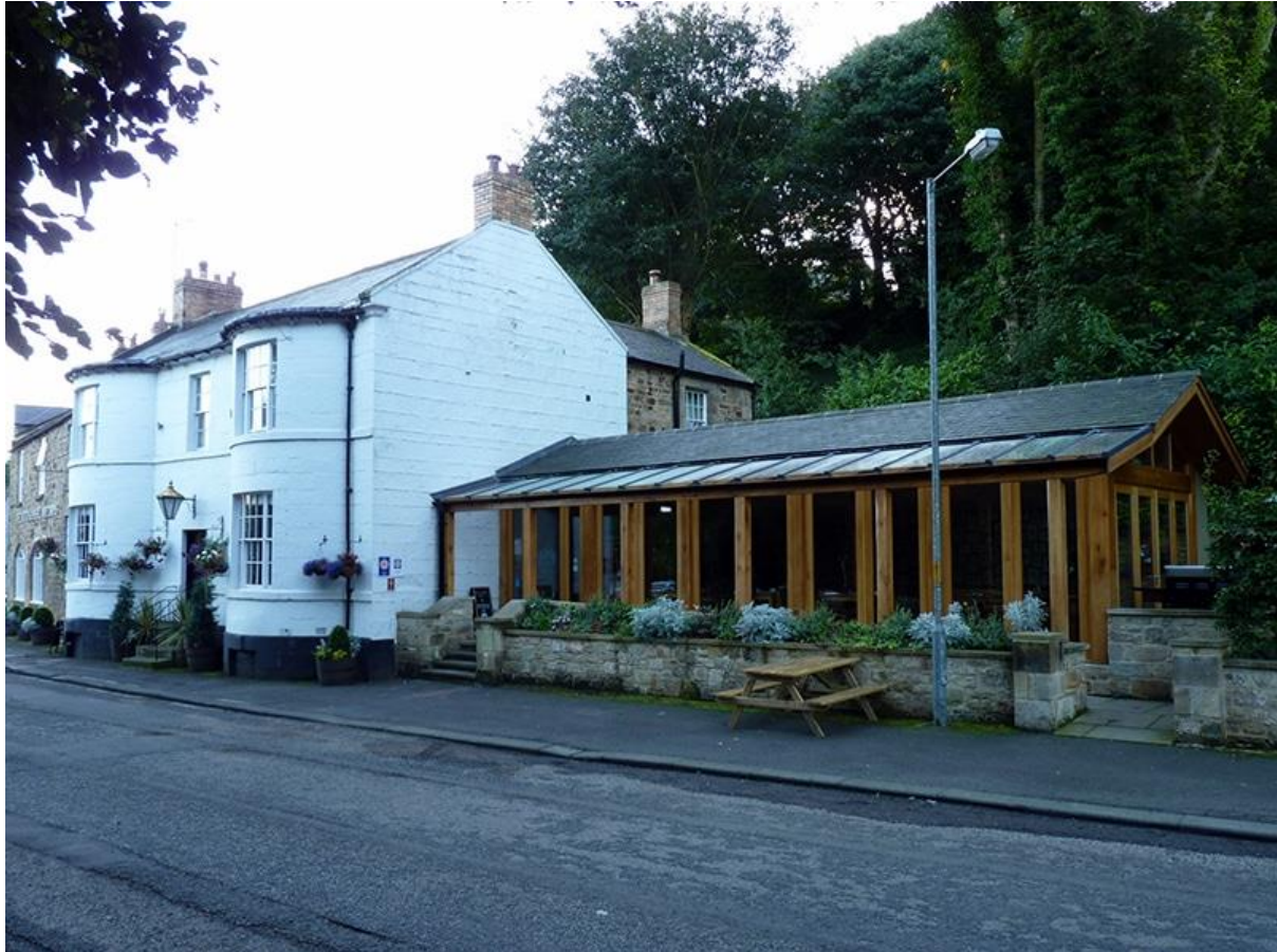
Image 6: View from south-west showing the current timber & slate function room extension
