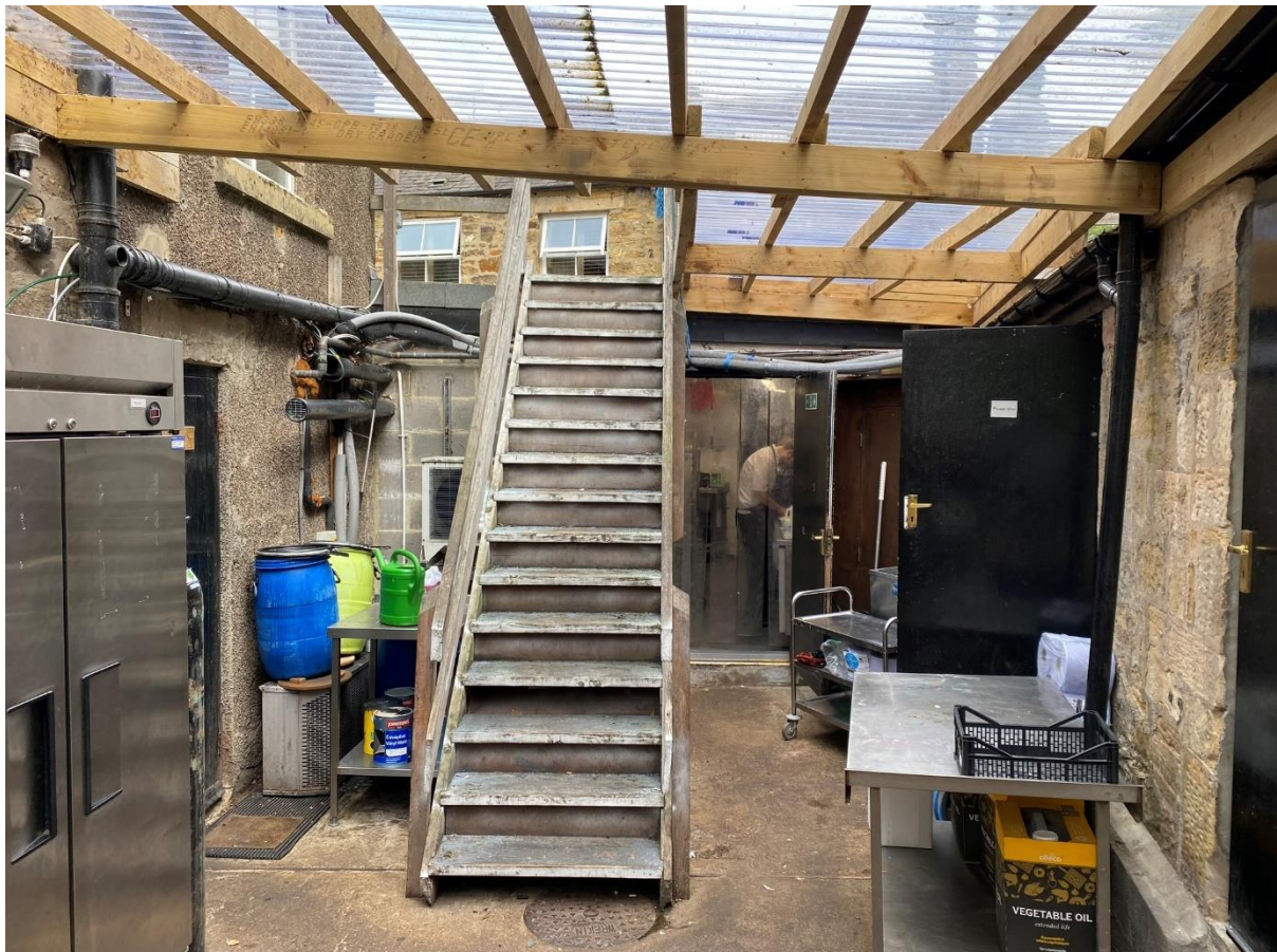
Image 13: Existing storage area
