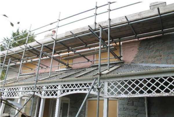
Plate 3: View of the (SW) long elevation
