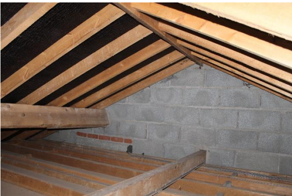
Plate 7: View of interior of the shallow kitchen loft void
