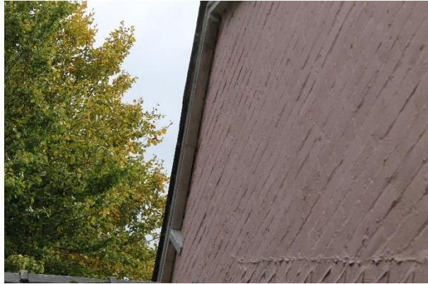
Plate 6: View of NE gable with timber soffits evident
