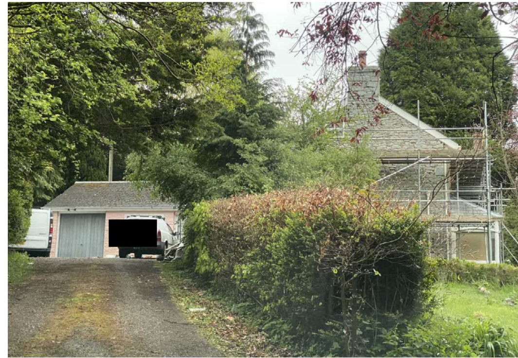
View from the driveway, towards the house
