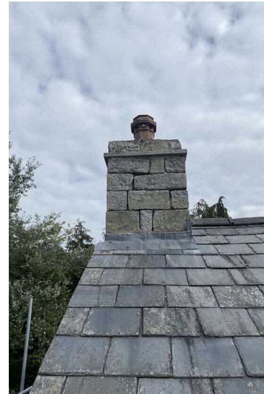
Existing slate tiled roof
