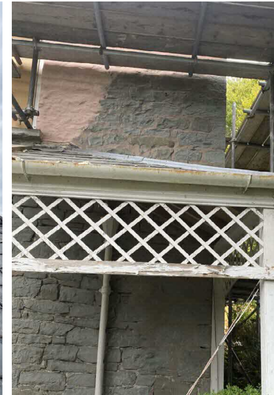
Existing stonework (front elevation) where paint has been removed
