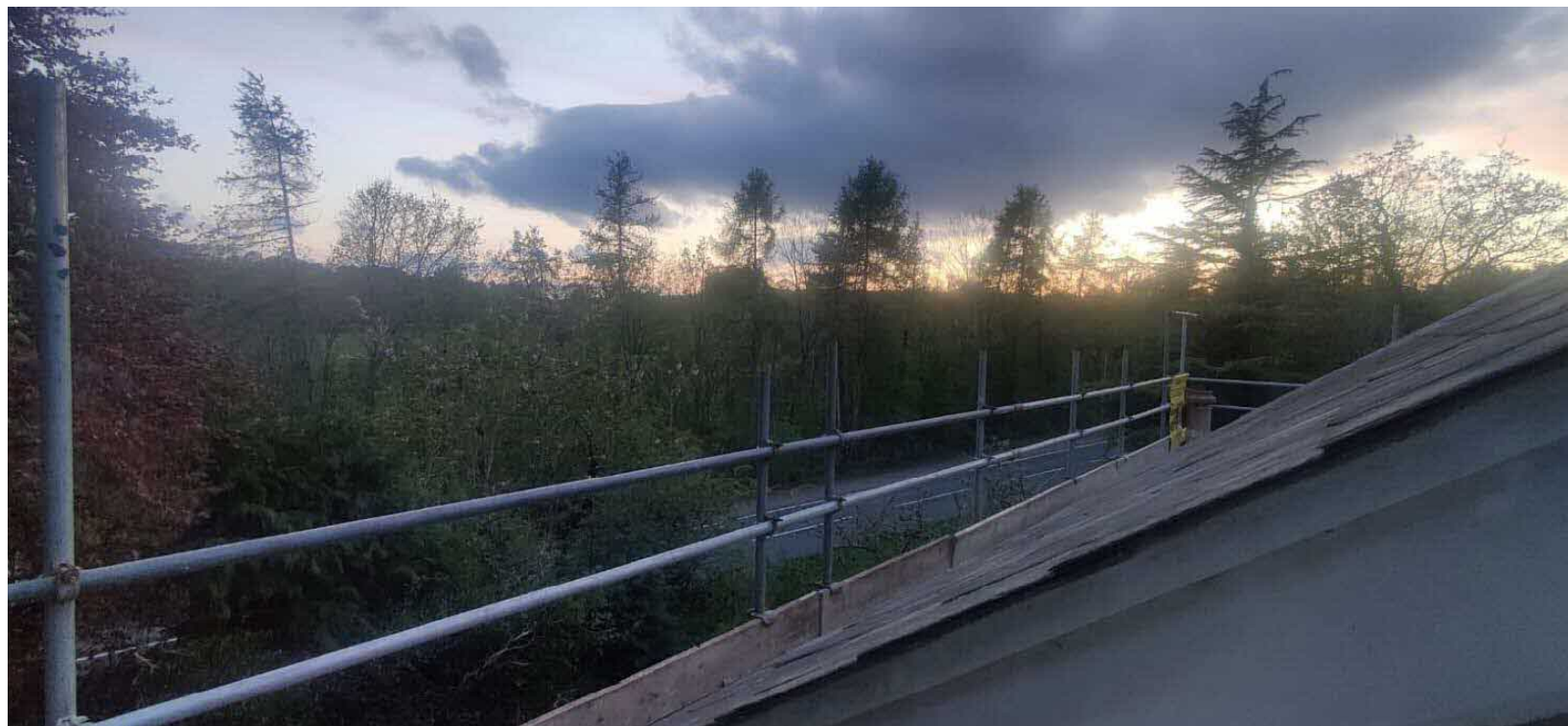
View from roof level, towards the River Wye
