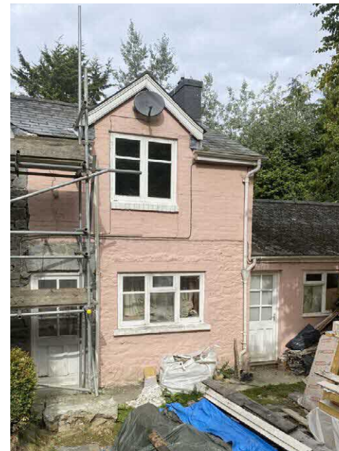
Existing outrigger/two-storey extension
