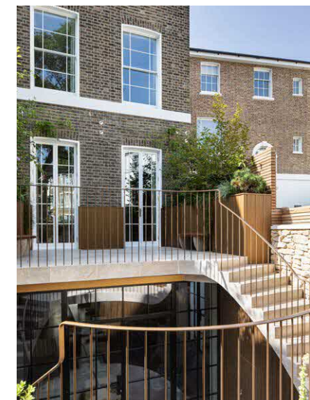
New extension to a Listed property within a Conservation Area in Camden
